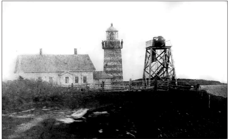
Early view of West Quoddy Head Light Station, probably in the mid- to late 1850s. Fog signal bell tower at right. Third order Fresnel lens installed in tower. Note the two keepers on the gallery. Photo courtesy of the U. S. Coast Guard.
