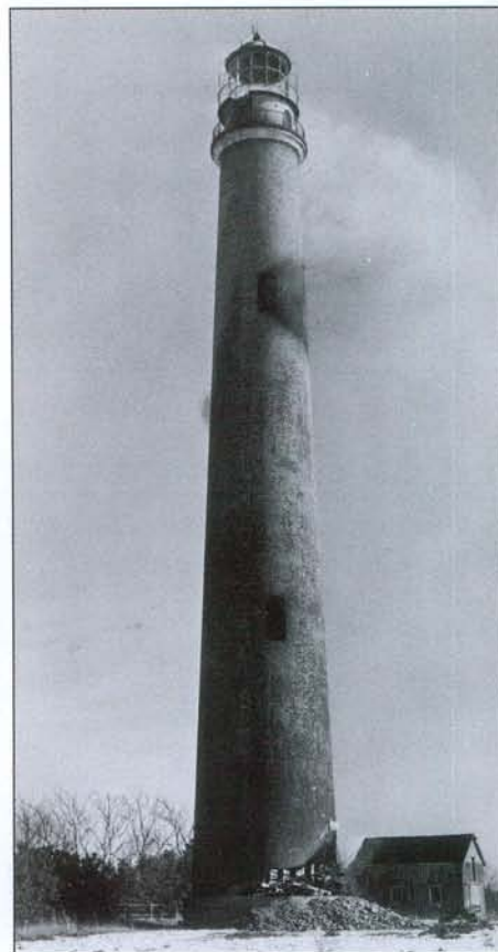
The tower acts like a chimney as smoke pours from windows and the lantern.
