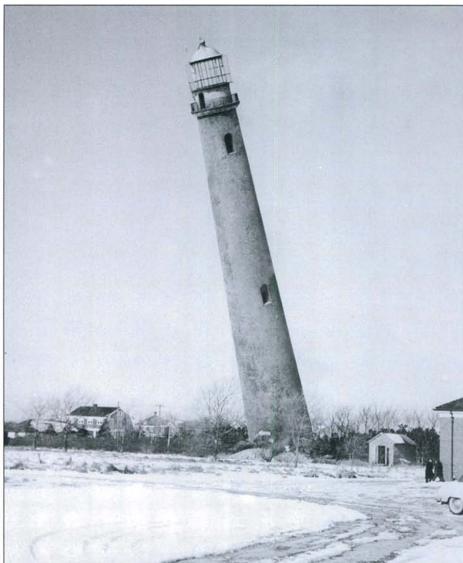
Going, going, gone! When the timbers burn through, the tower collapses to the beach, December 23, 1948. The building below is the Shinnecock Coast Guard Station boat house. Coast Guard photos courtesy of Al Penny.
