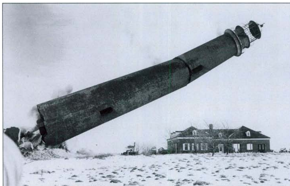
Going, going, gone! When the timbers burn through, the tower collapses to the beach, December 23, 1948. The building below is the Shinnecock Coast Guard Station boat house. Coast Guard photos courtesy of Al Penny.
