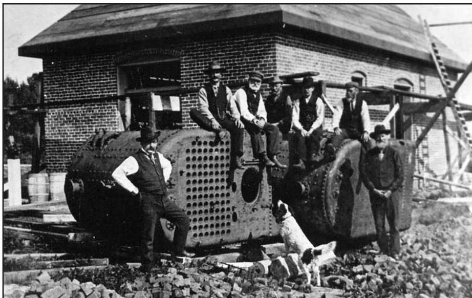
Above – Working on the chimney of the Seul Choix fog signal building. Note the two whistle fog signals on either side of the chimney. Photo courtesy of the author. Below – Workers install a boiler for a steam-powered fog signal. Lighthouse Society photo.
