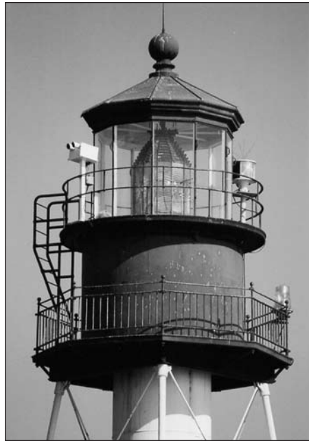
The 12-sided, 3rd order Fresnel lens can be clearly seen in the lantern room. The object at left is a fog detector. On the upper level at right is a Vega optic (made in New Zealand) which now serves as the primary optic at Point Loma. The lens on the lower level, at right, is a 300 mm standby, battery-powered optic. Photo courtesy of Kim Fahlen.
