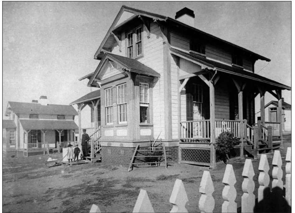
Top – Front of the east dwelling, with a keeper and kids on the front porch. The windows on the porch at right raise up into the wall and serve as doors. The dwelling design was used at San Luis Obispo and Table Bluff (Humboldt Bay). The picket fence in the foreground is a standard design used at many light stations.
