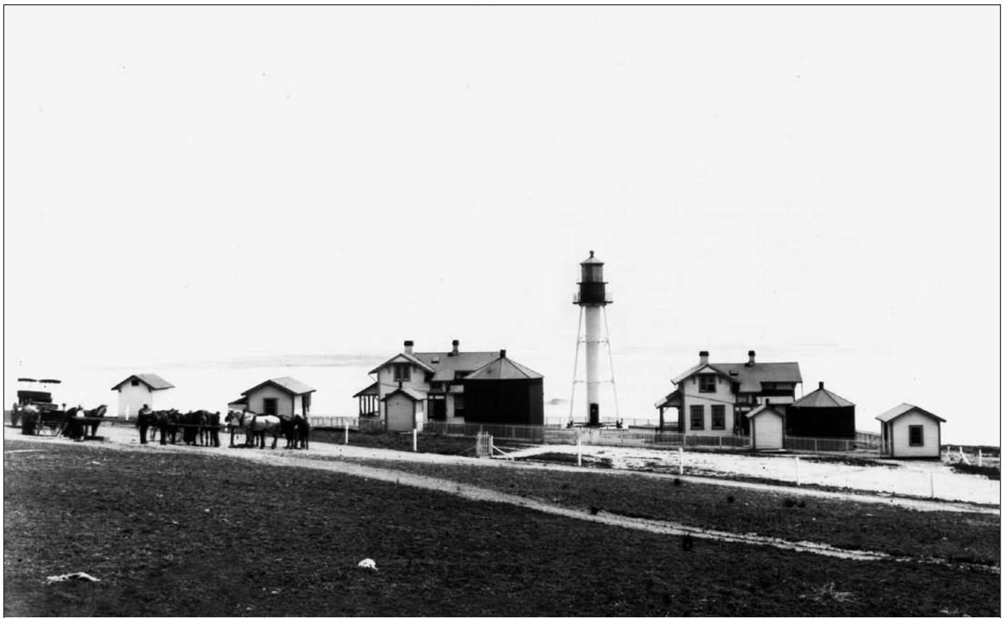
Point Loma Light Station, circa 1905, prior to the construction of the fog signal building. Workshop at right, small buildings are privies, and large cisterns at right of each dwelling. Note horses and wagon at left. Photo courtesy of the San Diego Historical Society.
