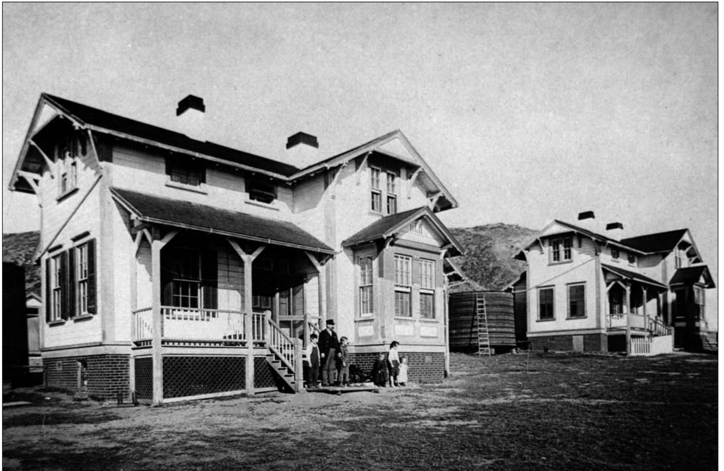
Bottom – The west dwelling with keeper and kids. The cistern for the east dwelling can be seen between the buildings, circa 1893. Both photos from the U.S. Lighthouse Society collection.
