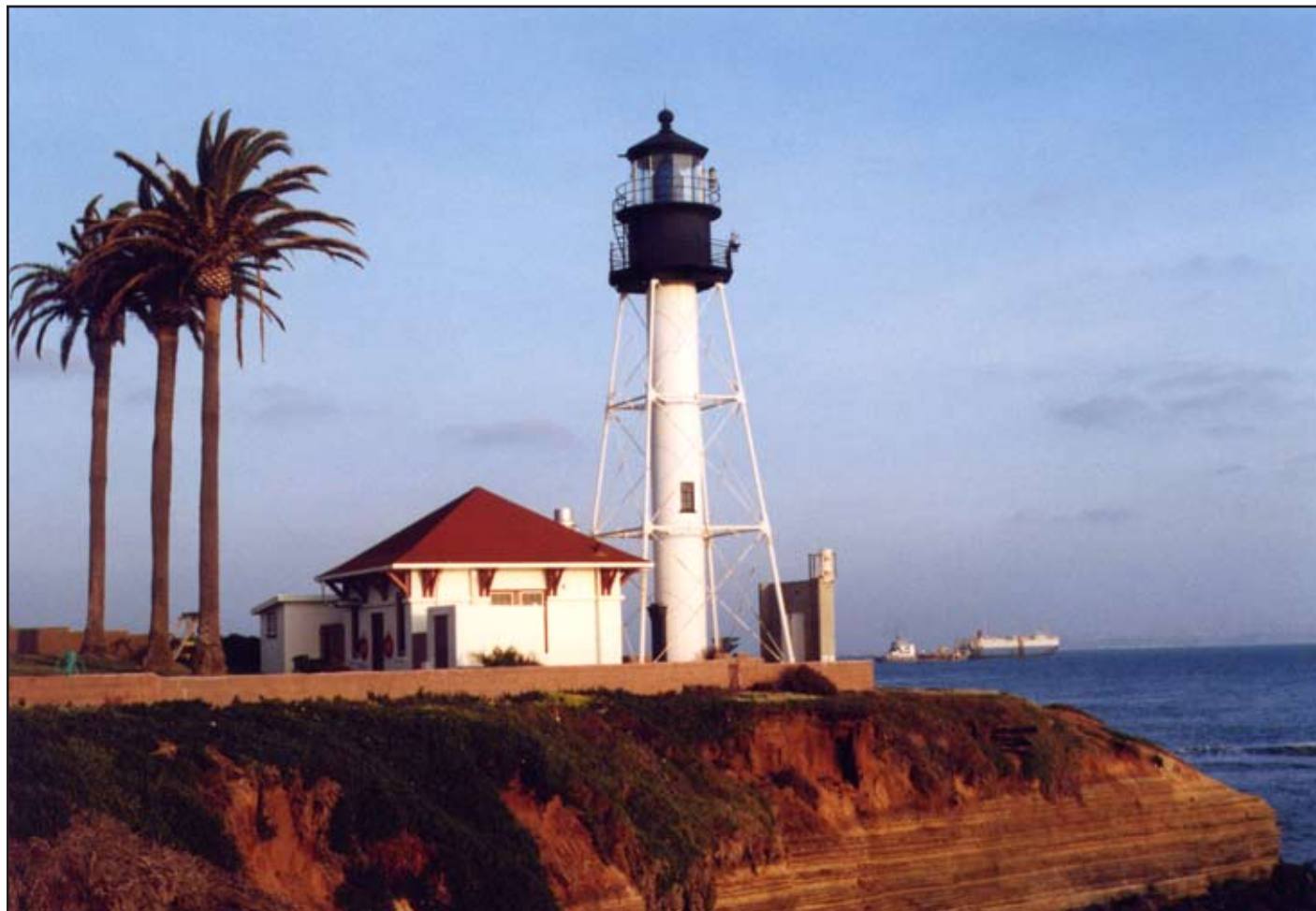
Point Loma, from the west, showing the fog signal building to the left of the tower and the modern electronic fog signal baffle, at right. Compare how close the bluff is to the tower with photos that appear later in this article. Photo by Kim Fahlen.
