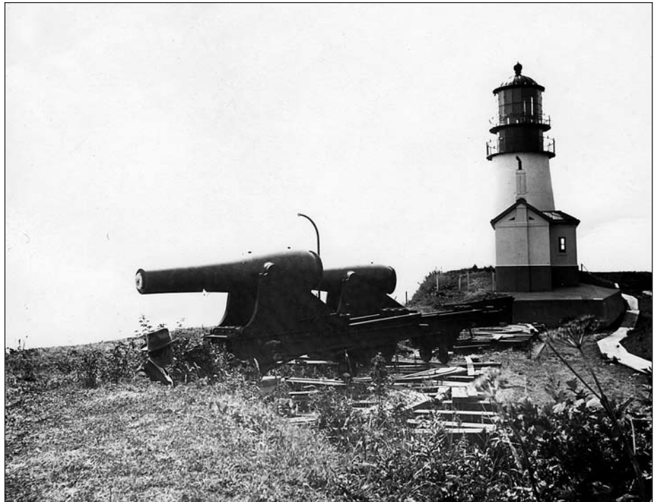
Right – 15-inch guns were installed near the Cape Disappointment tower sometime early in the 20th century, possibly during World War I. USLHS photo, date unknown.
