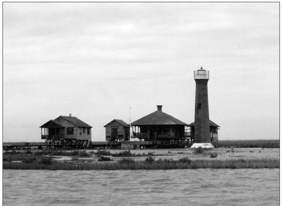
The Aransas Pass Light Station in 1995. From left, Assistant Keeper's dwelling, store house, Head Keeper's house and tower. Photo by Ainsley Dixon.
