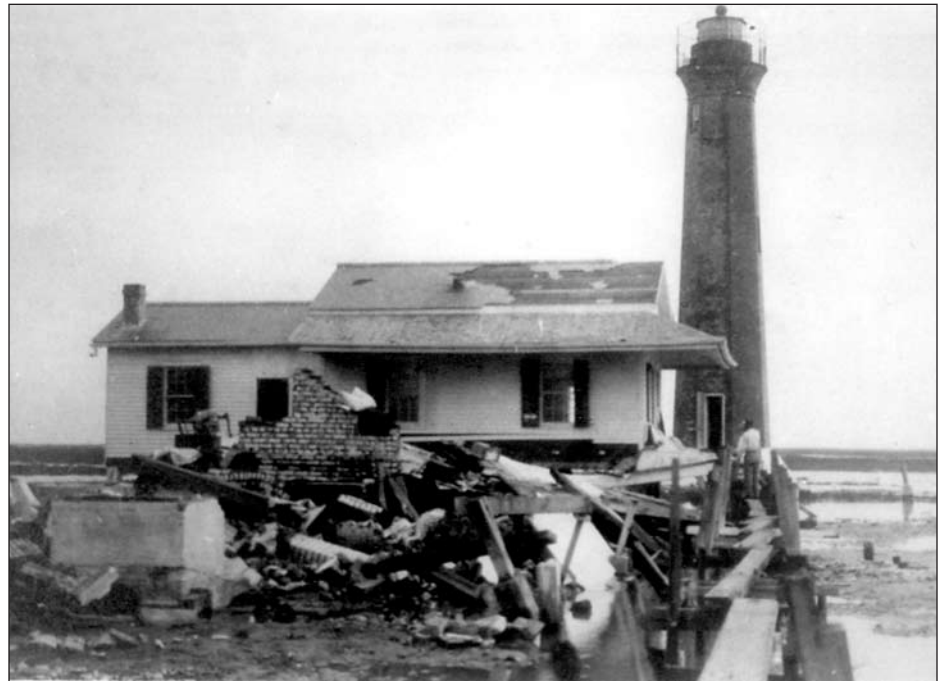
Above – The damaged Assistant Keeper's dwelling after the 1917 hurricane.
