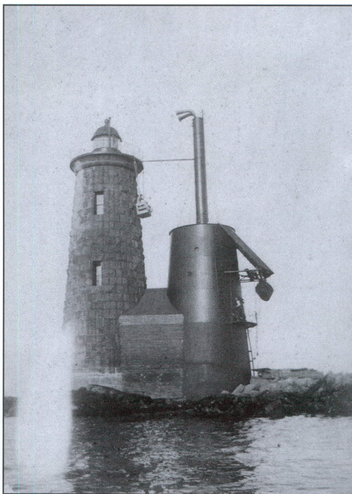
The 1871 Whaleback tower with a fog signal building, left; the fog signal horns are located at the top of the smoke stack. Note the keeper in a basket alongside the tower, probably repointing the stone. A dory hangs from davits at left. Hazel Sargent photo.
