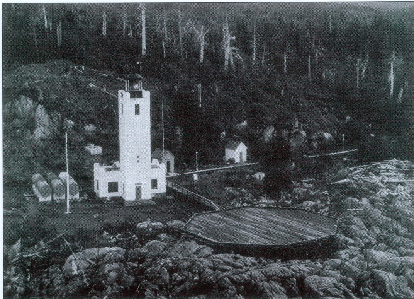
When the station was automated the Coast Guard installed the helicopter platform in the foreground to bring in servicing personnel. Oil storage tanks, at left, were used to fuel the continuously-running generators. They have since been removed and the aid solar powered. Photo courtesy U. S. Coast Guard.
