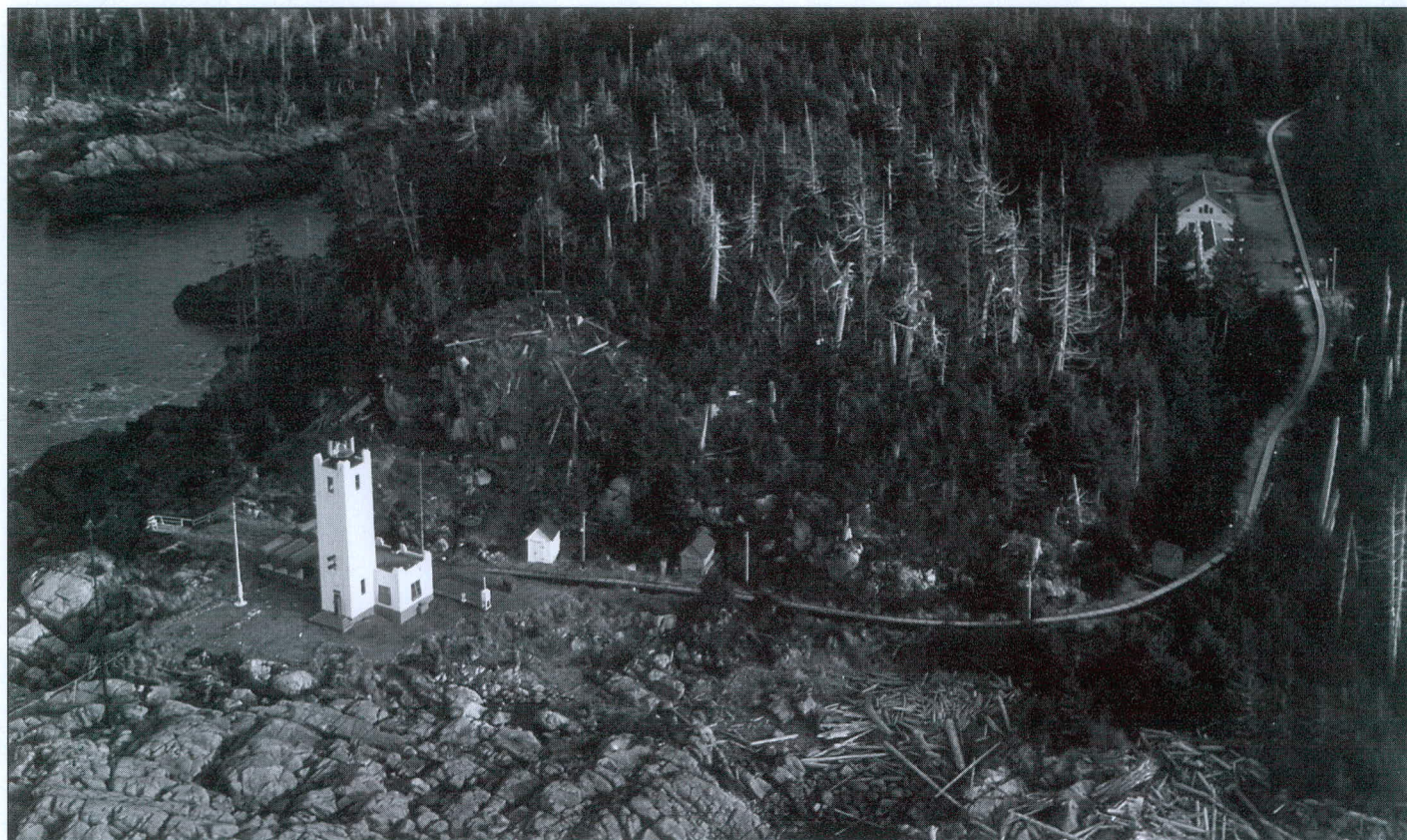
Tree Point Light Station in 1963 showing the new tower and the railway which runs past the dwellings (top right) and to the lagoon with the landing dock and crane. Photo courtesy U. S. Coast Guard.
