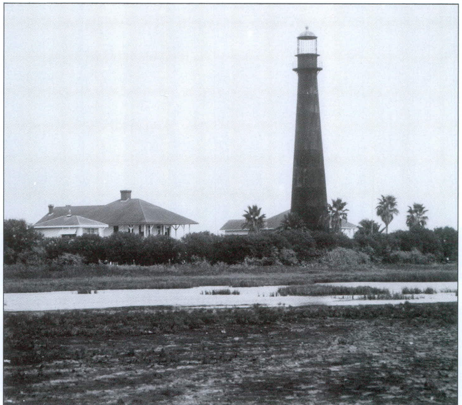
Bolivar Point Lighthouse established in 1852. The 95 foot high cast iron tower was completely dismantled by Confederate forces during the war. Photo by Randy Chase.
