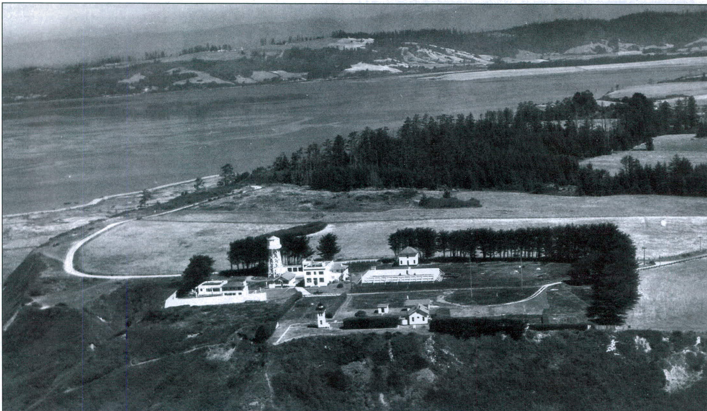
The Table Bluff Light Station circa 1970. The tower, sans dwelling at left, oil house and fog signal building. The duplex has been removed. Buildings in the background are World War II Navy structures. Lower Humboldt Bay in the far background. U. S. Coast Guard photo.
