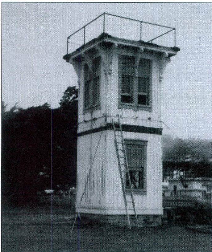
Above – The Table Bluff tower being dismantled. After the lantern was removed the tower was cut in half in the area at the top of the ladder. Ray Glavich photo 1982.
