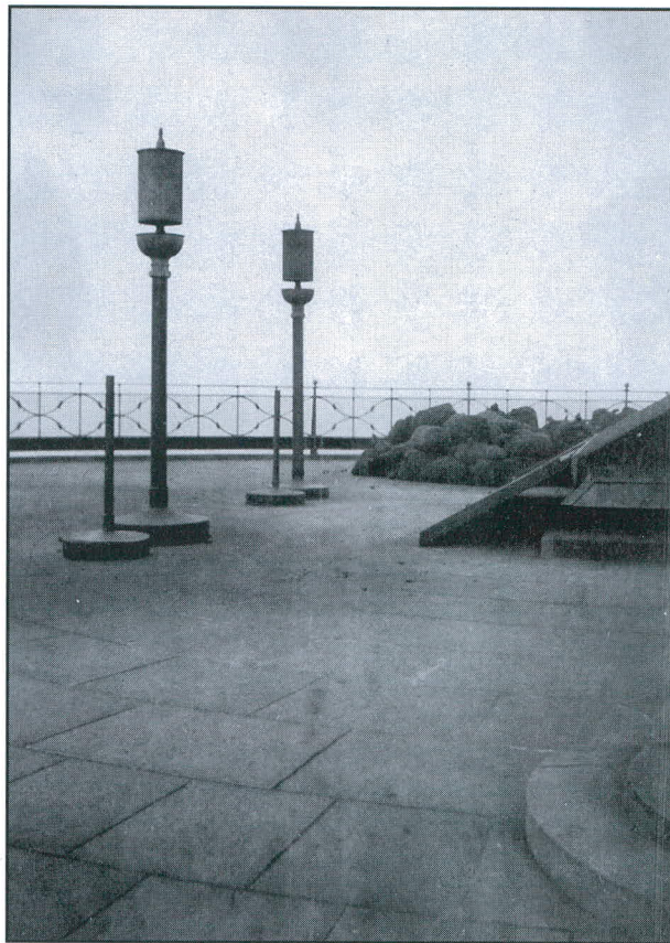
The original sound (fog) signal at the lighthouse was a steam-powered whistle, shown above in duplicate. The deck of the caisson was used to collect water which was funneled into a cistern in the caisson. U. S. Lighthouse Society photo.
