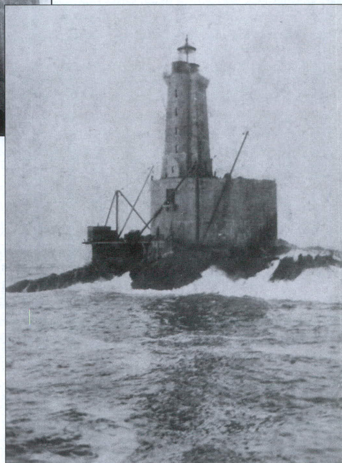
Above – 1891 photo of the completion of the tower on the caisson. Structure at lower left is the barracks which replaced the barracks vessel. This structure was often inundated during storms.
