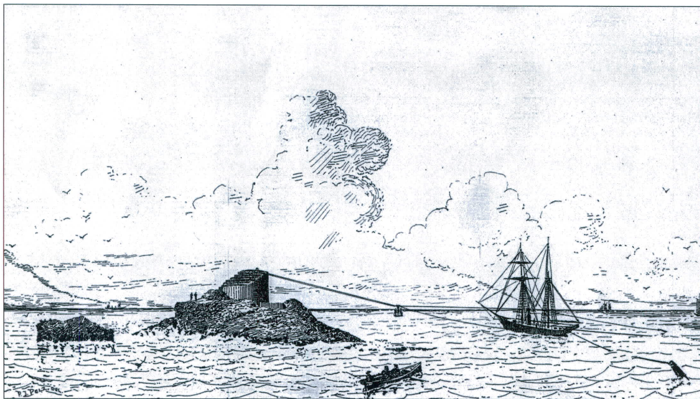
Men traveled between the barracks ship ( La Ninfa and later Sparrow ) on a platform and "clothes Line" type of rig. Drawing from the 1884 Report to Congress from the Lighthouse Board.
