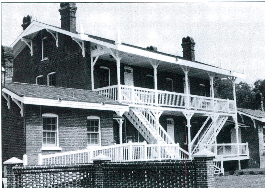
The restored duplex keeper's quarters. The low additions at left & right are the kitchens. Note the elaborate veranda. Photo by Dan Spinella.
