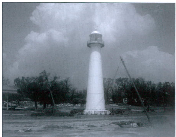
Biloxi Lighthouse in August 2005 right after Hurricane Katrina. Photo by City of Biloxi.
