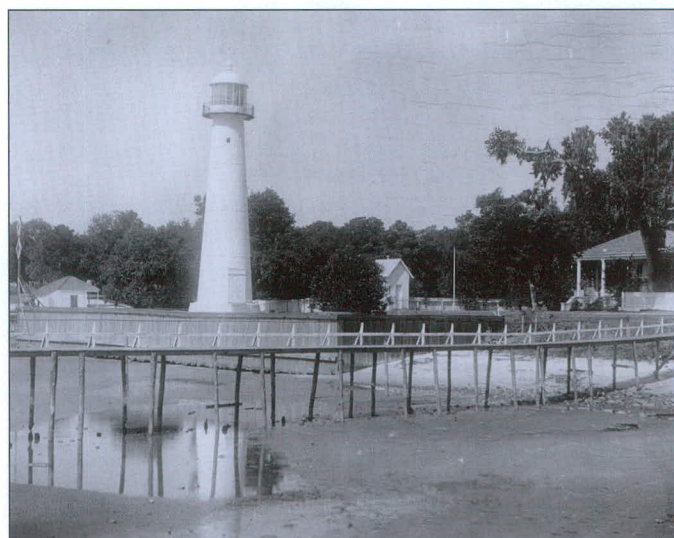
The Biloxi Lighthouse in 1892. U.S. Coast Guard photo.
