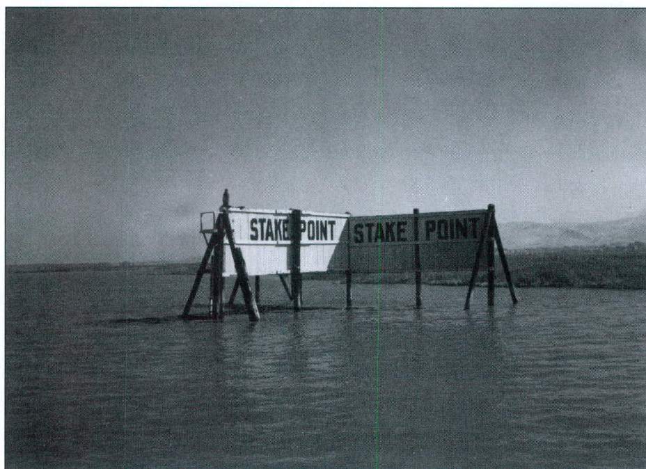
Top-Stake Point Light and sounding board in the Sacramento Delta. Sounding boards like this echoed a ship's whistle and provided direction and distance in the fog, prior to arrival of radar. A minor oil lamp can be seen at the left end of the "T"'s stem. USLHS photo.
