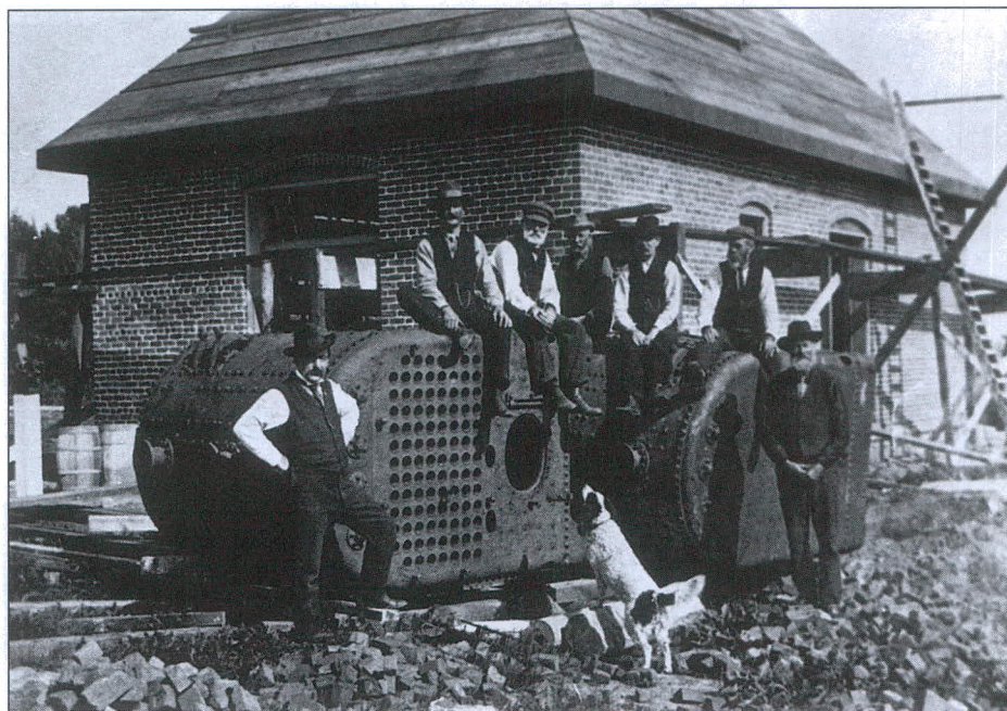
The workmen who constructed the new fog signal building pose for the camera against the steam boilers for the new fog signal. Note the roof of the fog signal building hasn't been shingled in this 1903 photo. Photo courtesy of the Apostle Islands National Seashore.
