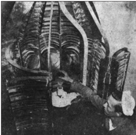
Below – Coast Guardsman changing the lamp in the Third Order Fresnel lens. Photos courtesy of Ponce de Leon Inlet Lighthouse Preservation Association.
