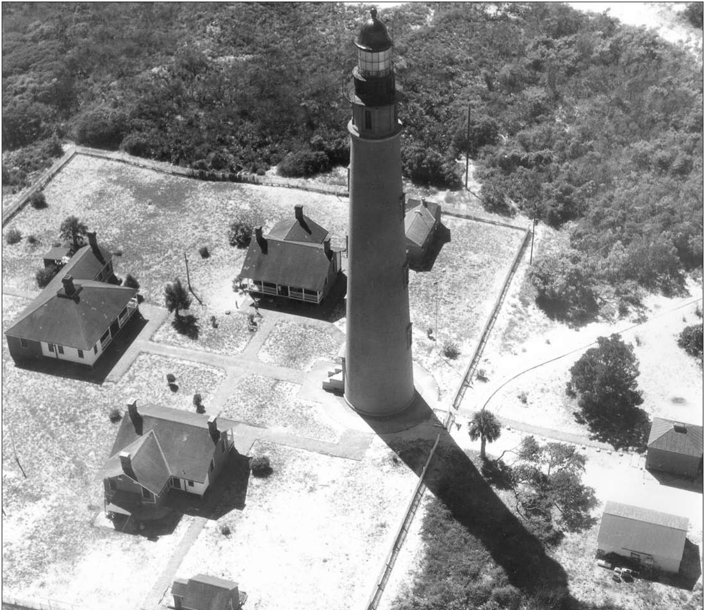
Post World War II view of the Ponce de Leon Inlet Light Station: Starting at the left center is the principal keeper's dwelling. The assistant keeper houses are between this and the tower. Each dwelling has a privy/woodshed located behind it. The small structure attached to the principal keeper's kitchen is a laundry shed. The privy is at a little distance from the house, and you can see a walkway but not the privy itself. The first assistant's privy/woodshed, partly hidden by the tower, was enlarged in 1943 to accommodate the radiobeacon equipment. The building at the right with the ventilator on the roof is the oil house. The other structure nearby was a garage which has since been torn down. Photo courtesy of U. S. Coast Guard circa 1951.
