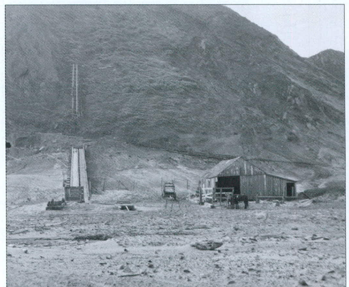
Right—The old horse barn just before removal, probably about 1907. Notice the new road cutting across behind the barn and the remains of the old east side tramway and stairs at left. USLHS photo.
