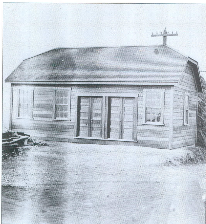
The carpenter-blacksmith shop circa 1890. Above the roof on the right side is a call bell pole. A keeper on watch could ring up his relief or call the head keeper if he had a problem. USLHS photo.
