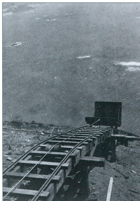
Below—The ocean side tramway with the car being lowered (some 280 feet) for another load of Texaco kerosene. Circa 1900. USLHS photos.
