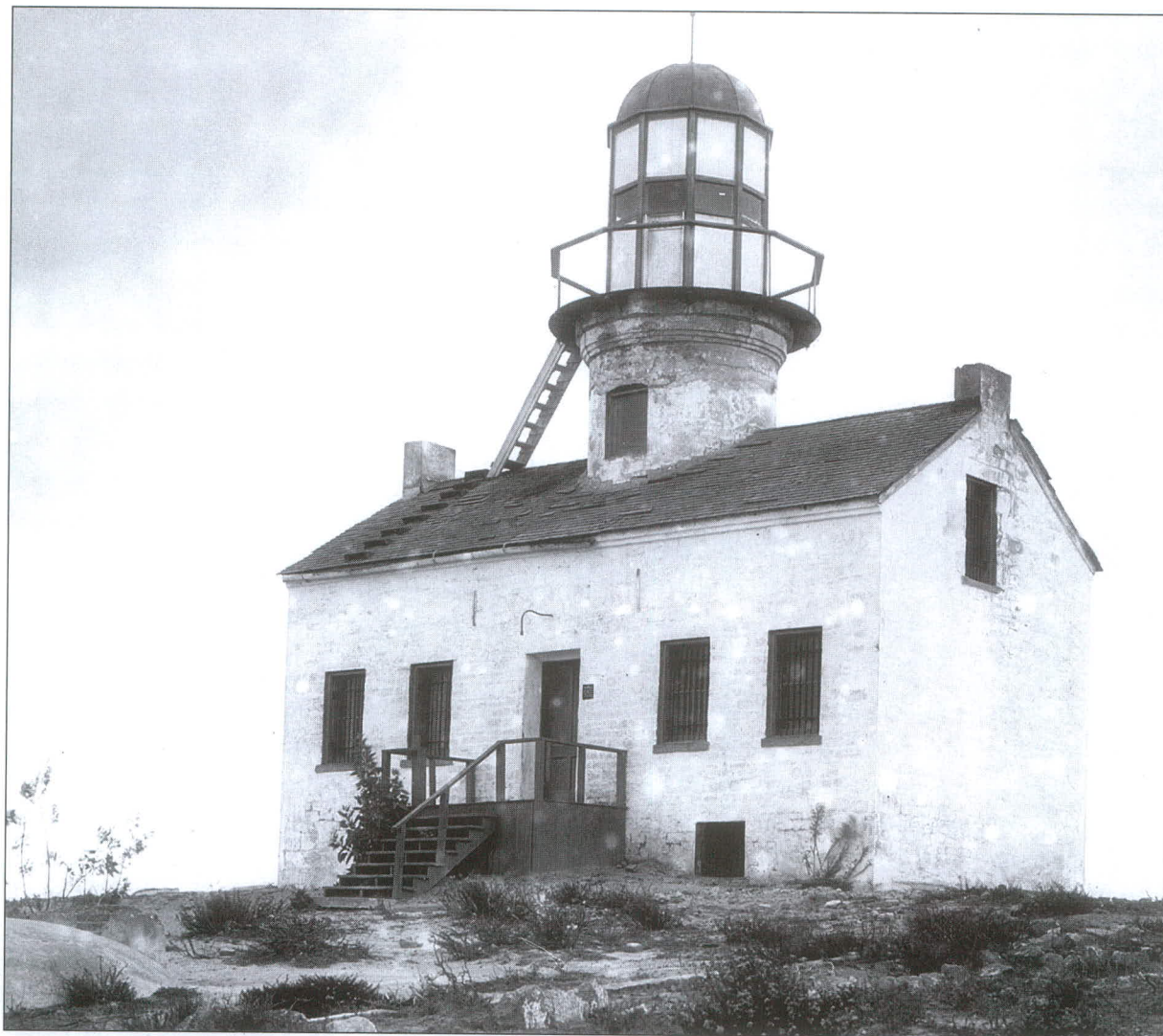
Point Loma circa 1931 showing the windows installed in the lantern room by the Army. Photograph courtesy of the U. S. Lighthouse Society archives.
