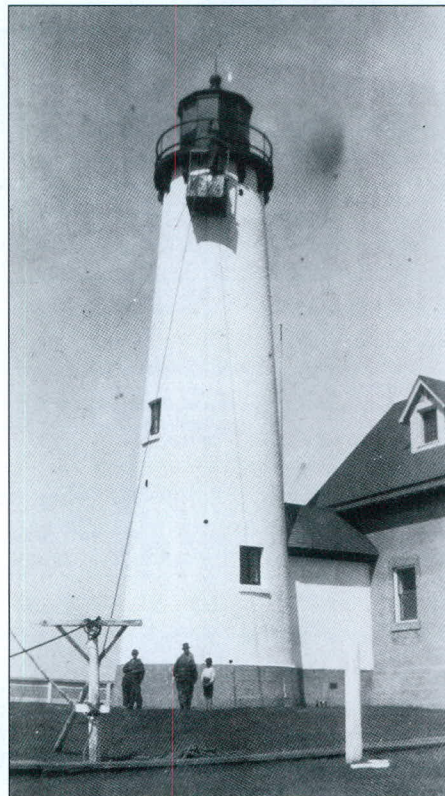
The keeper painting the tower by means of a bos'n chair. Photo courtesy of Betty Bacon.
