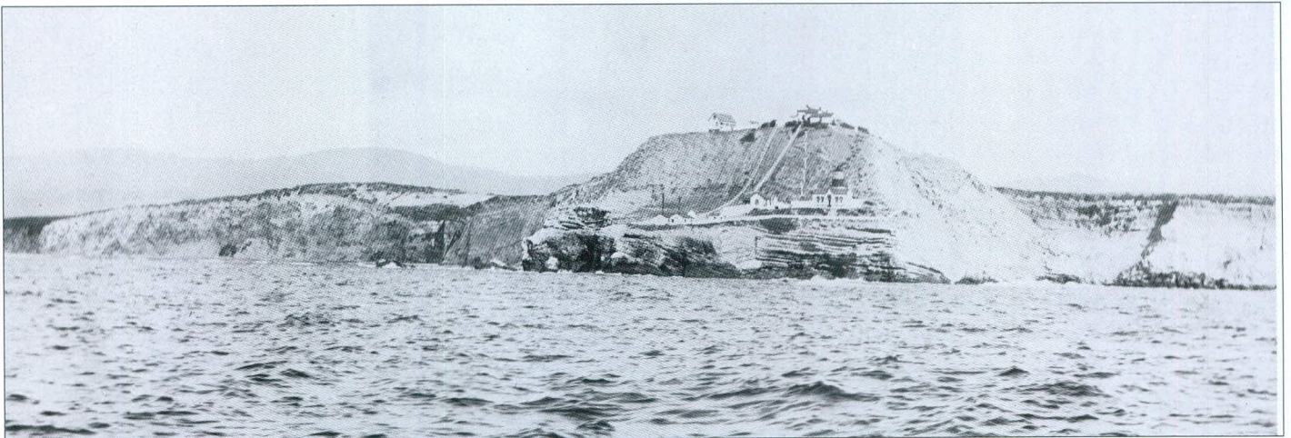
The remote bleakness of Point Conception is all too evident in this turn of the century photo. The original two peaked roof fog signal building is at left. The house that would be the Owen's home for 4 years, and later blocked by the new fog signal building, can be seen at the base of the staircase. The telephone poles marching up the hill behind the tower carried the wires for the bell call signal system between all the keepers' homes. National Maritime Museum photo.
