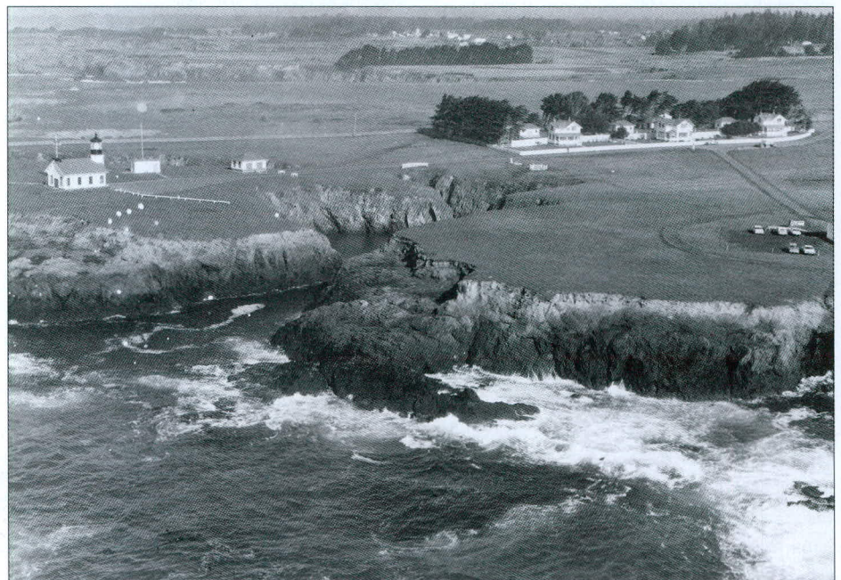
In the middle of the photo an arm of the sea almost reaches the road. The erosion from the north stops just short of the carpenter-blacksmith shop. The head keeper's house is in the middle. U.S. Lighthouse Society photo.
