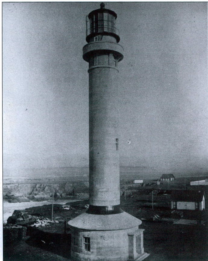
Above – A supporting concrete 'donut' in place around the base of the tower and the lantern is finished, but lens not installed.
