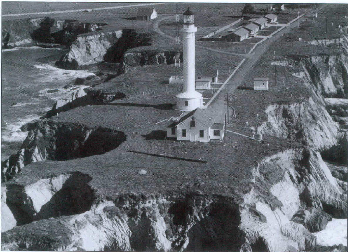
Point Arena Light Station looking east in the 1960's. The badly eroding cliffs have eroded even more since this photo was taken some 30 years ago. The original fog signal building was 125 feet west of the present structure (foreground). The four houses replaced the 1907 bungalows in the 1960s. The barn top left, has been removed. Official U.S. Coast Guard photo.
