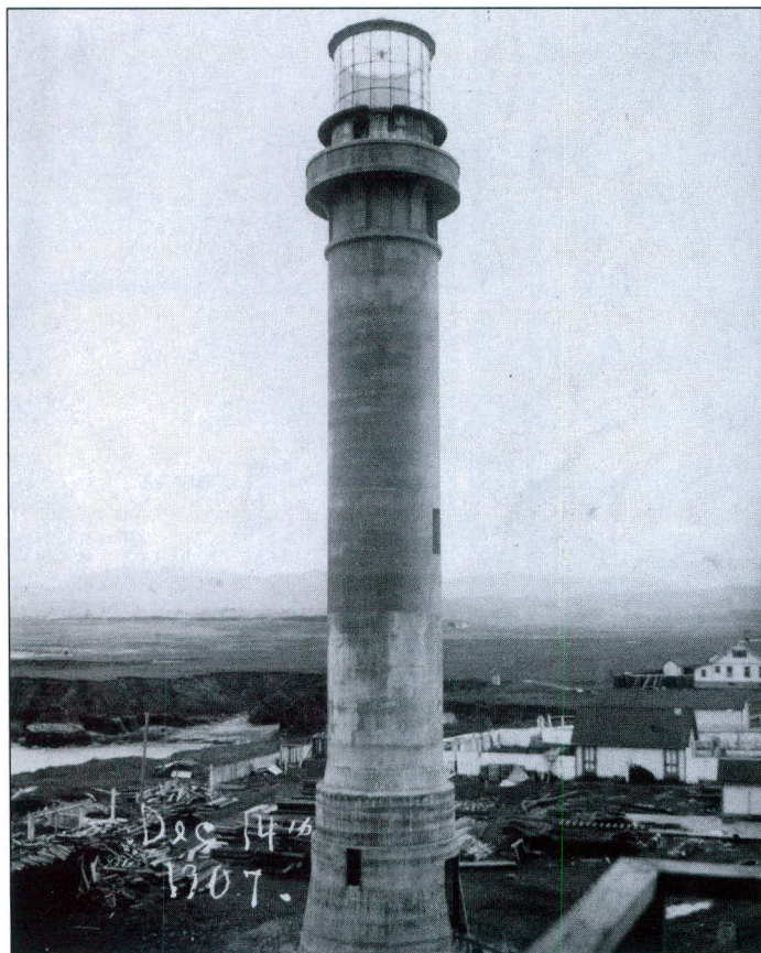
Above – Dec. 14, 1907 – The scaffolding removed and a portion of the lantern installed. One of the new keeper's bungalows can be seen far right.
