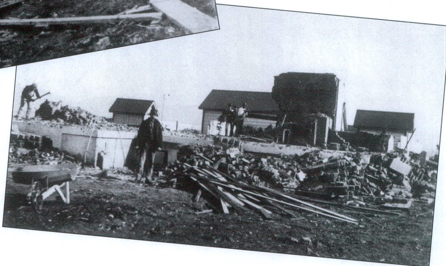
Below – The remains of the fourplex with wooden storage sheds in the background that survived the quake. All U.S. Lighthouse Society photos.
