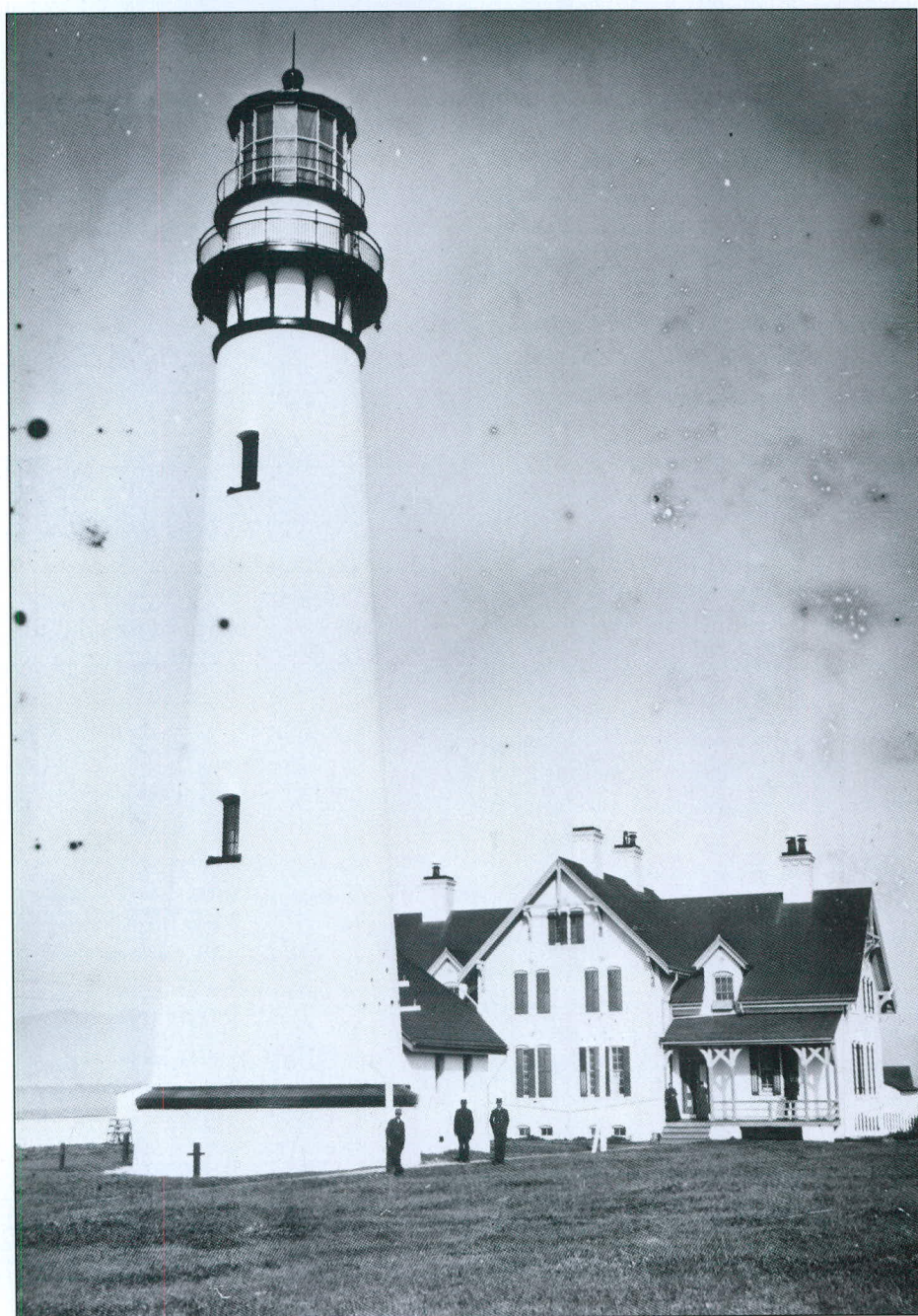
The original Point Arena tower and brick fourplex, constructed in 1870, were badly damaged in the 1906 earthquake and had to be razed. This tower design was used at Pigeon Point, CA, Cape Hatteras, NC, Sand Island, AL and several other locations around the country. National Maritime Museum photo.
