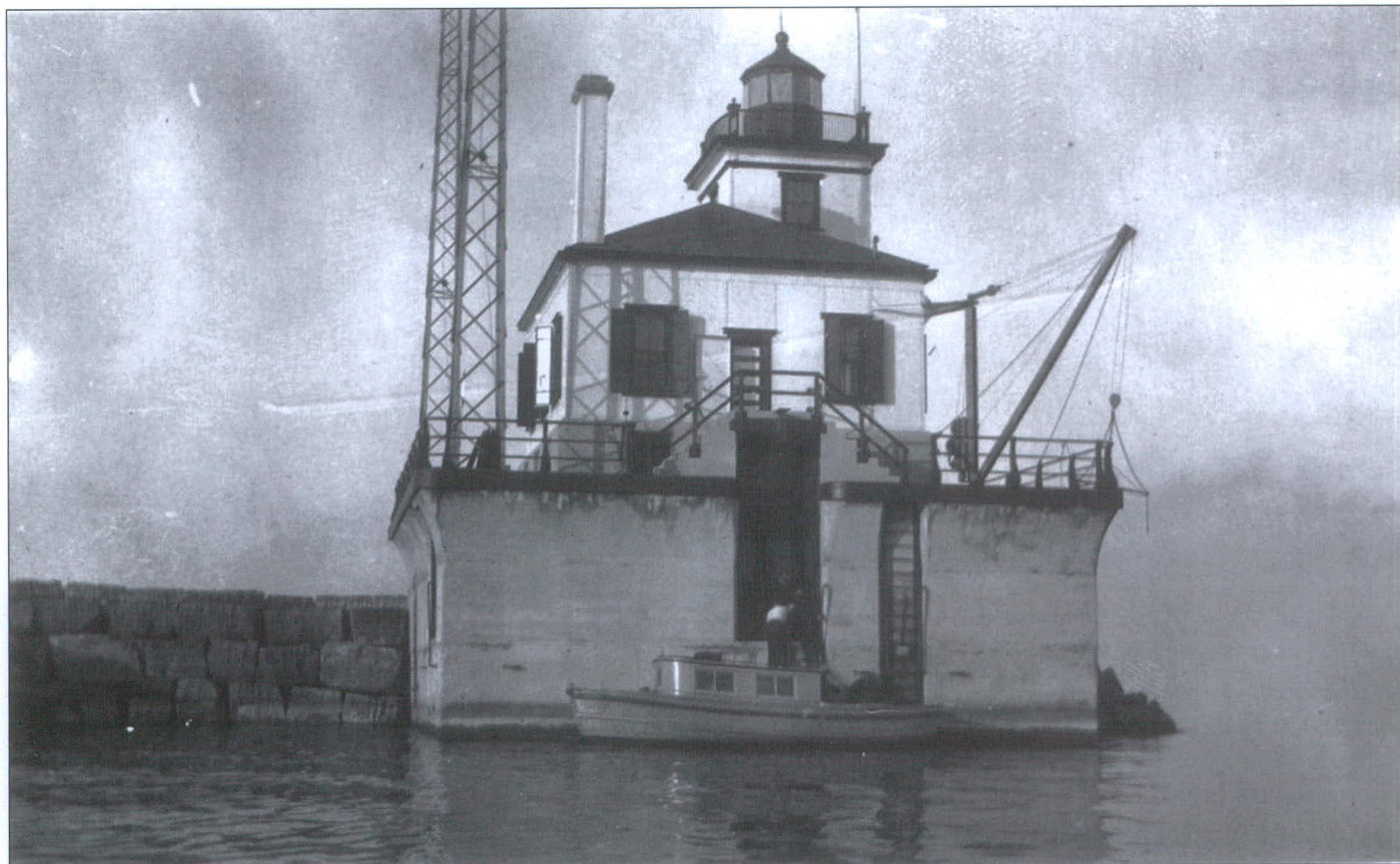
Circa late 1930s, the lighthouse launch is alongside the south side of the caisson at the large equipment door into the basement machinery room. The two radio beacon antenna towers have been added on the west side of the caisson and a derrick on the southeast corner. Photo courtesy Bob Gode and H. Lee White Marine Museum.
