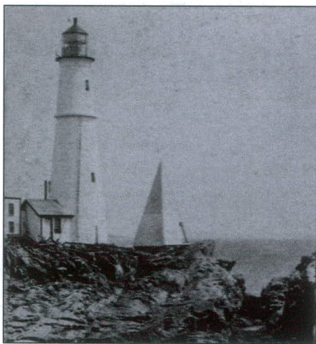
Portland Head Lighthouse, the first constructed under the Ninth Act. Note the vent atop the lantern. Pyramid shaped bell house at right. From an 1870 stereopticon card courtesy of Tim Carr.
