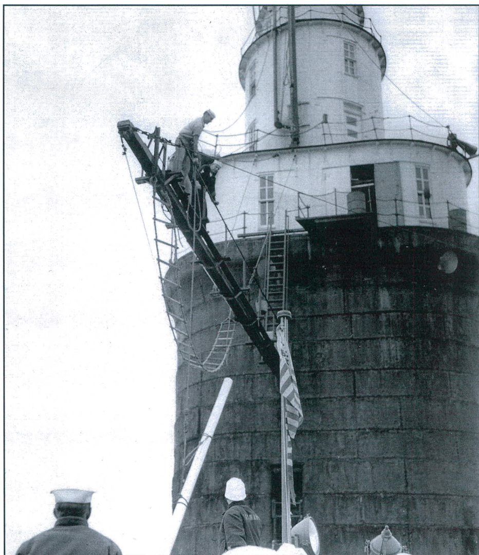
Coast Guardsmen on one of the two landing booms dropping a line to the supply vessel. The rope "Jacobs" ladder will be lowered to allow the relief crew to board the station. U. S. Lighthouse Society photo.
