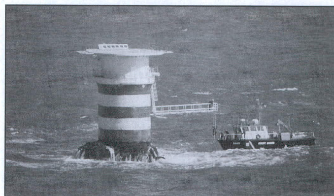
Right – In the early 1980s the caisson was painted with orange and white stripes to increase visibility in fog. Flood lights were installed under the flight deck. In this photo a solar array can be seen on the flight deck. A Coast Guard aids to navigation vessel is about to land service personnel. A 1990 photo by Sandra Shanklin.
