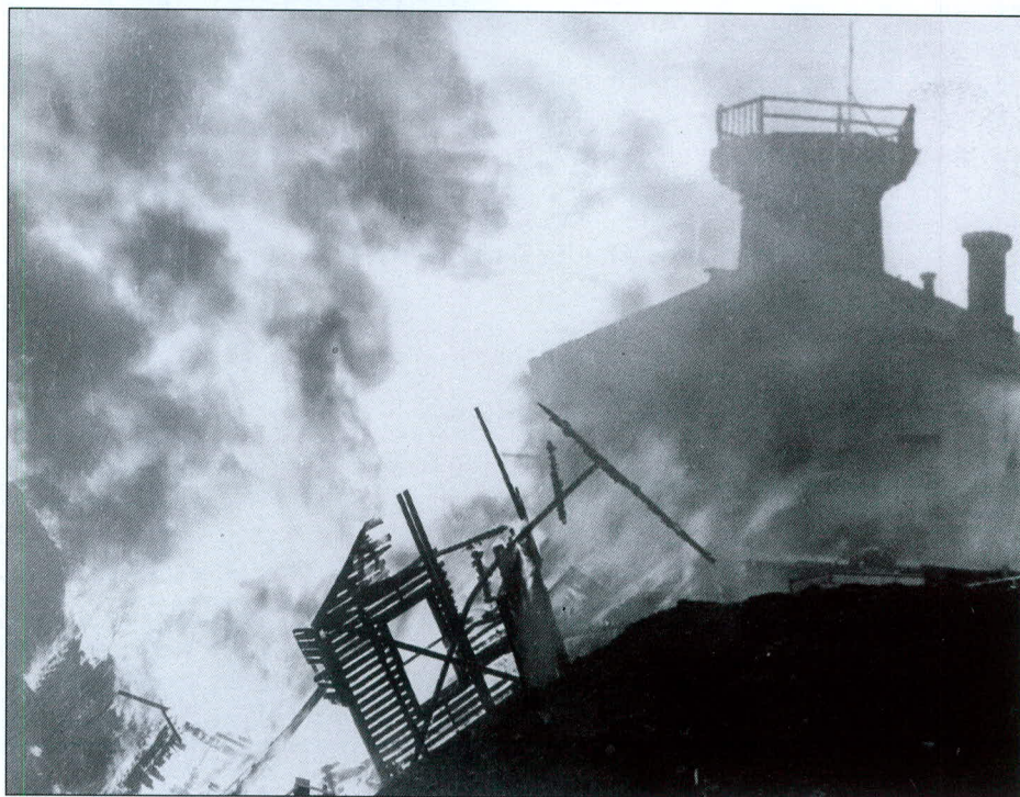
Below – Once the new Cape Hinchinbrook tower was completed the old structure was burned. Both photos courtesy of the U.S. Coast Guard.
