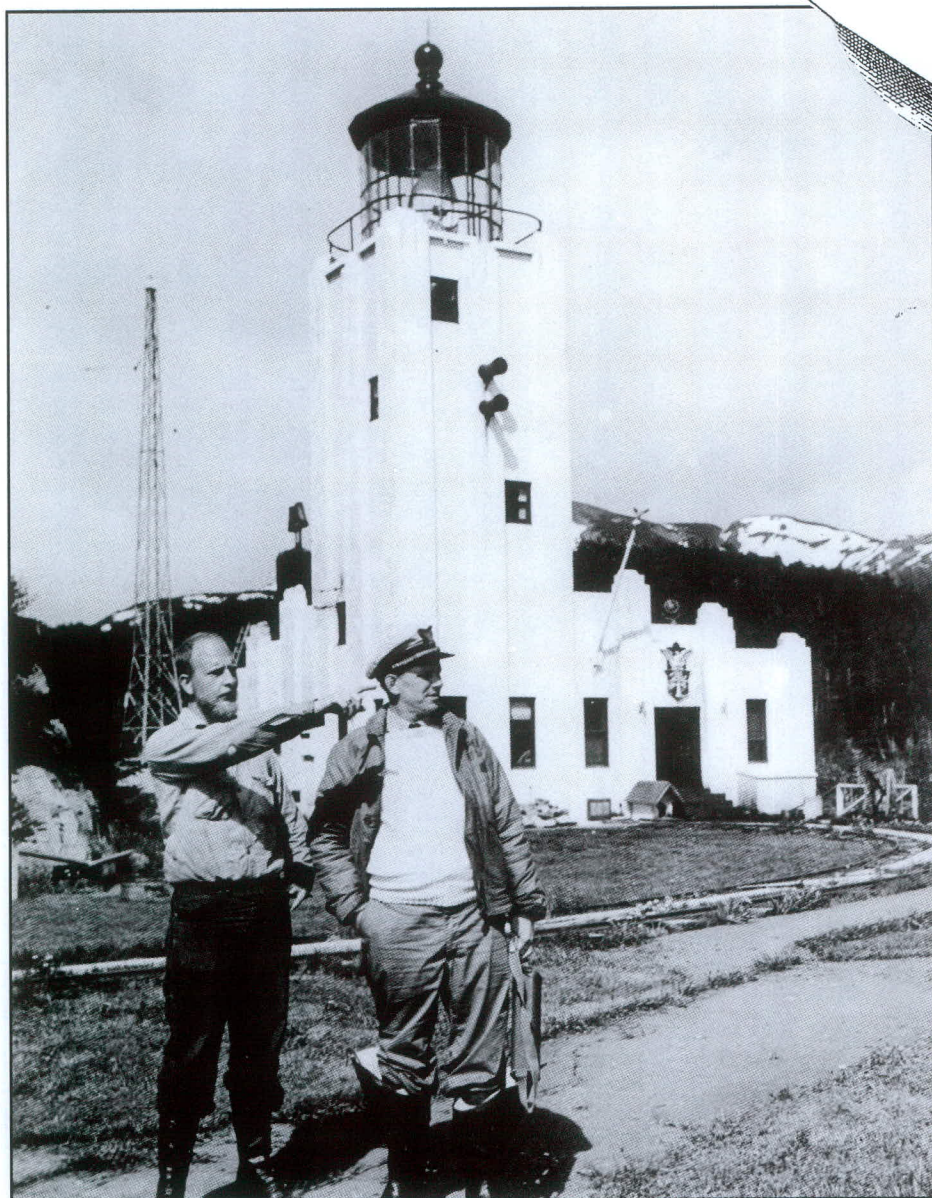
Cape Hinchinbrook Light Station when it was manned. Note the diaphone fog signal horns protruding from the tower and the old Lighthouse Service emblem over the entrance door. U.S. Coast Guard photo.
