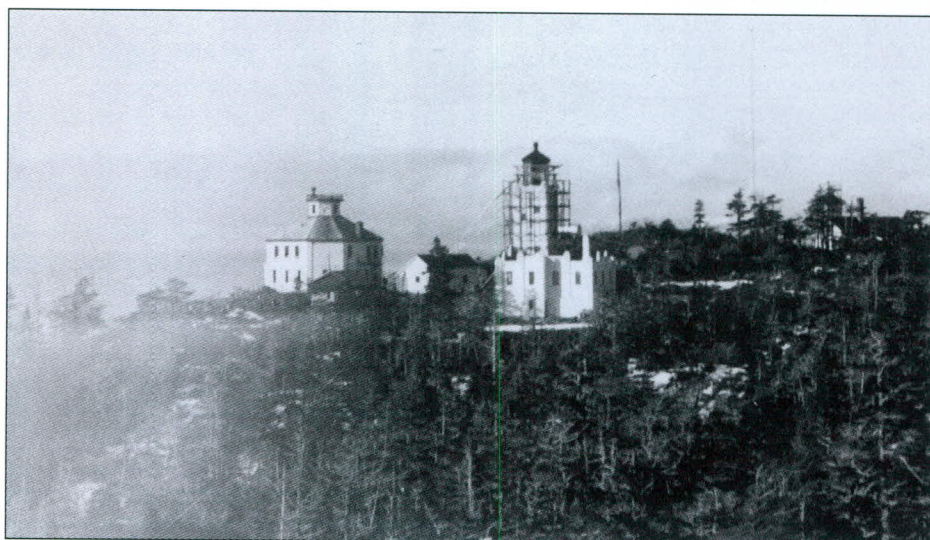
Left – The new Cape Hinchinbrook tower under construction in 1935. The old tower can be seen at left. The lantern of the old tower was used on the new building.
