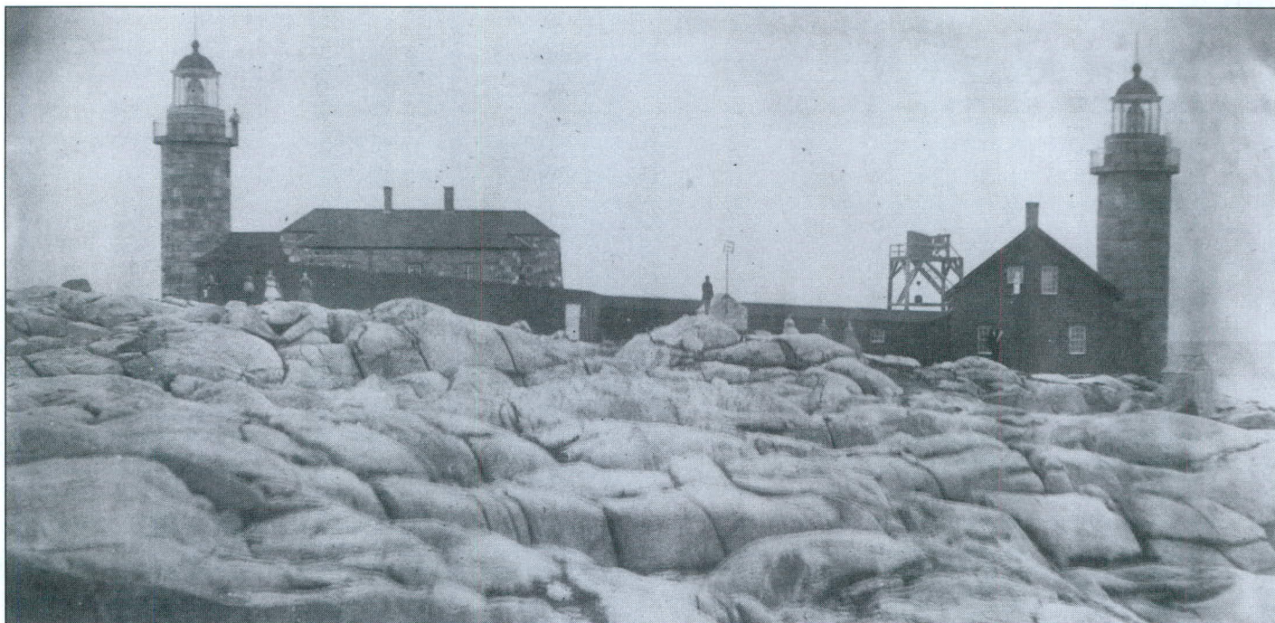
Matinicus circa 1860's. The structure in back of the right dwelling is the bell fog signal platform. Note the station personnel. It appears that the children are standing by the left tower, Keeper in the center and Keeper's wives to the right of him. U.S. Coast Guard photo.
