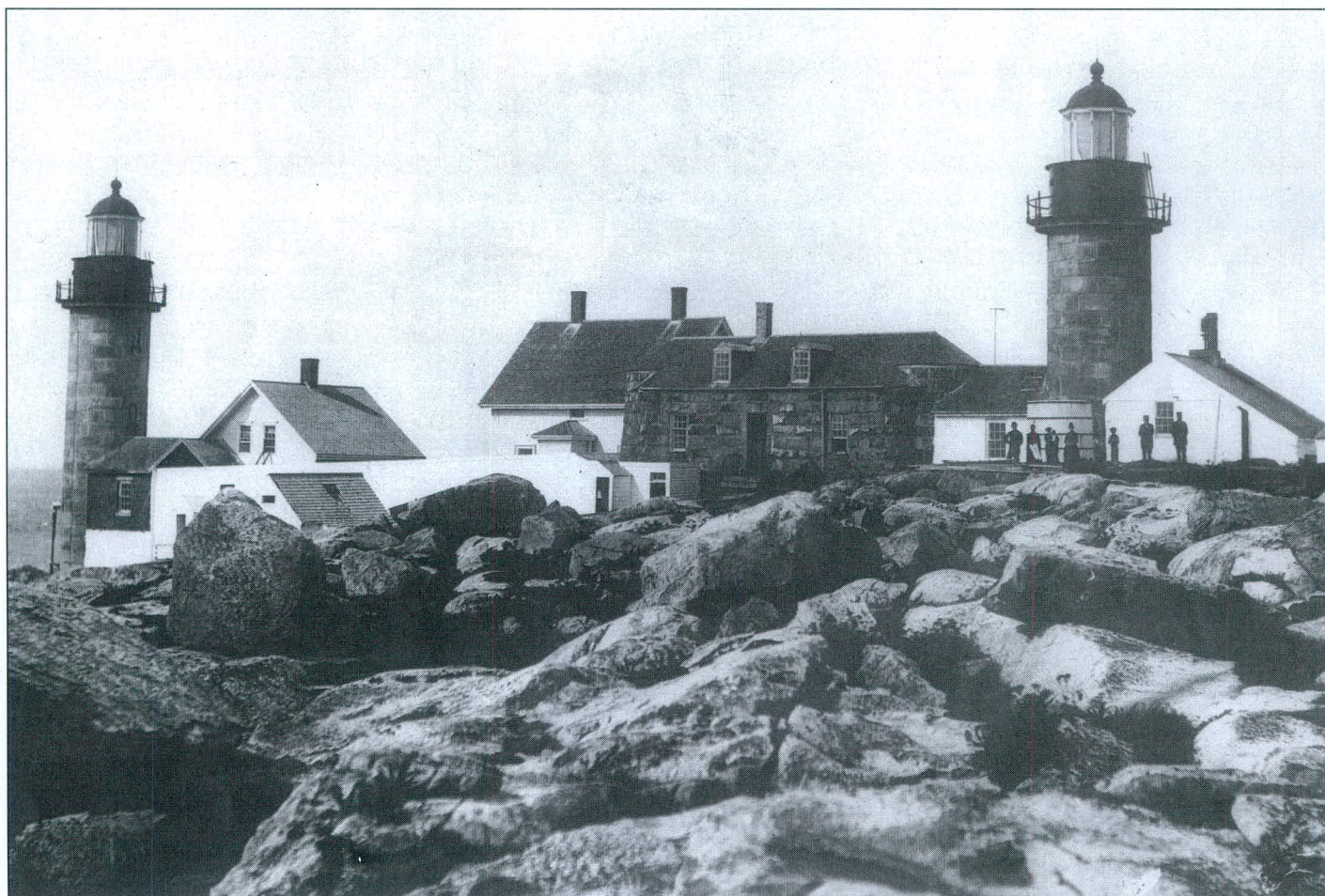
Matinicus Rock Light Station after construction of the 1857 towers, and after 1884 as the keepers in the photos are wearing uniforms. Note the original combination dwelling and towers just to the left of the right tower. The old towers have been reduced and incorporated into the roof line of the dwelling. The structure next to the right tower is the fog signal building. In this era the signal was a steam powered whistle. National Archives photo.
