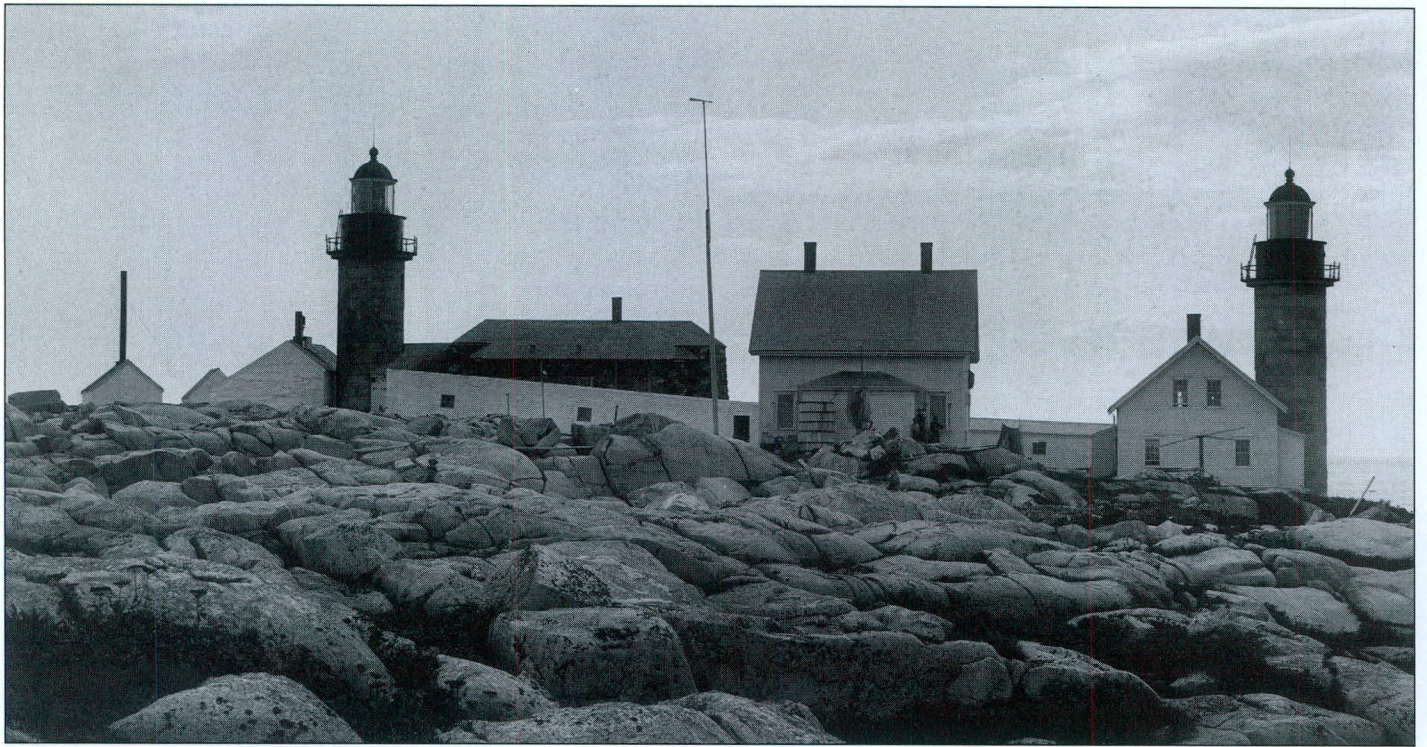
Matinicus Rock Light Station in the 1890's. From left — boathouse, fog signal building, tower, old stone house, keeper's house, assistant keeper's dwelling, tower. Note the covered walkway between the towers. Photo courtesy of the U.S. Coast Guard.
