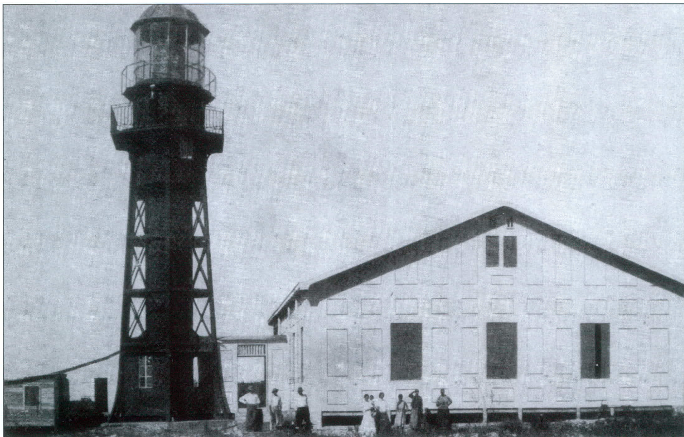
The completed Mona Island lighthouse. Most of the cast iron parts of this station were found on the beach by the American forces after the Spanish-American War. Except for the reconstruction of the San Juan tower, this station and that on Cabras Island are the only light stations constructed by the American government. Library of Congress photo.
