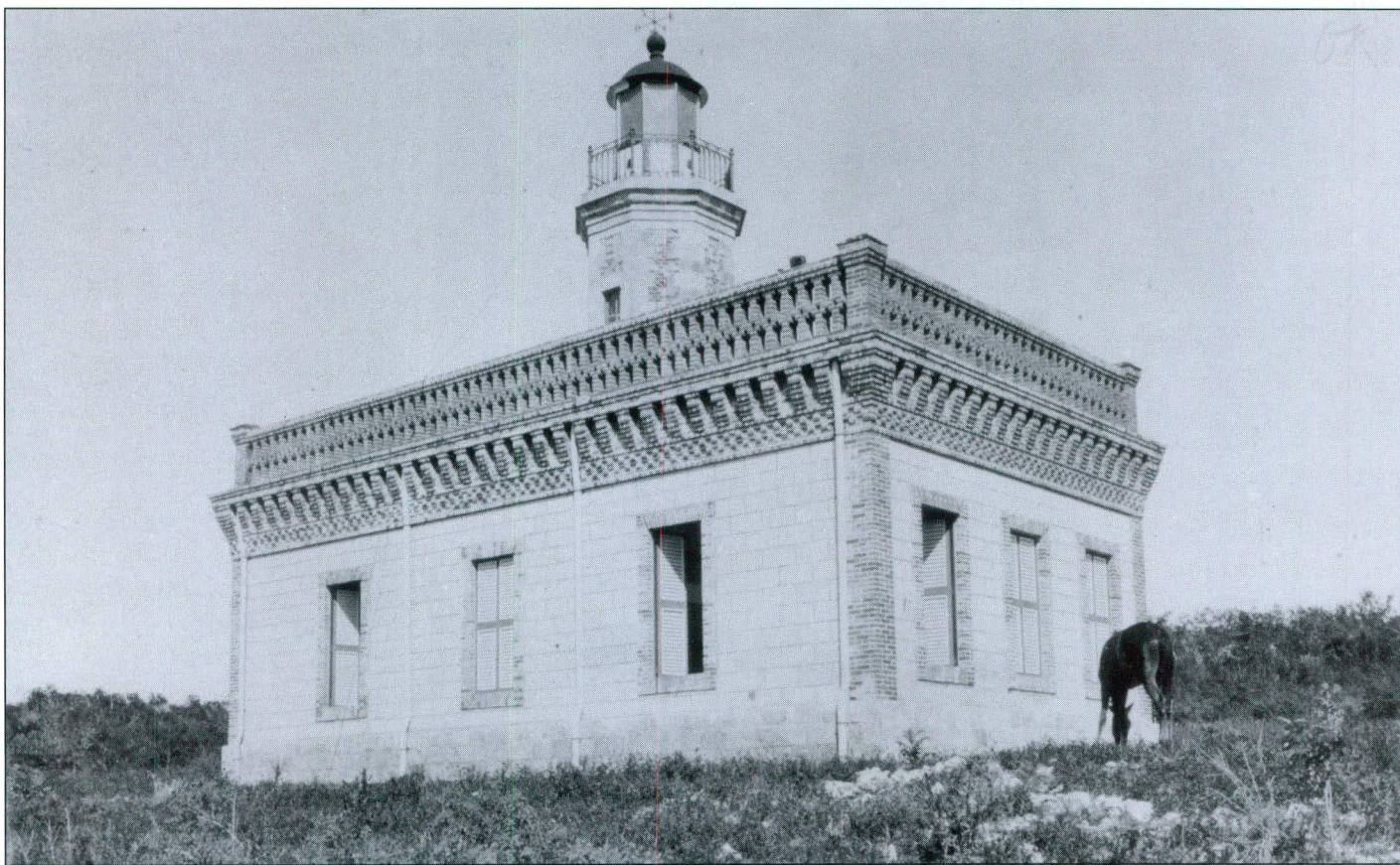
The unique Guanica Lighthouse, constructed in 1893, is located on the south shore of Puerto Rico midway between Cape Rojo and the City of Ponce. National Archives photo.
