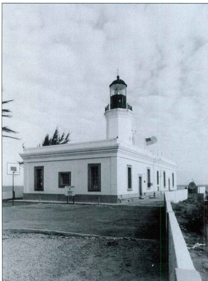
Point Figuras (or Pt. Figuero) was constructed in 1893 on the south shore of Puerto Rico and is typical of most PR lighthouses with a duplex quarters surmounted by the tower. Circa 1955, U.S. Coast Guard photo.
