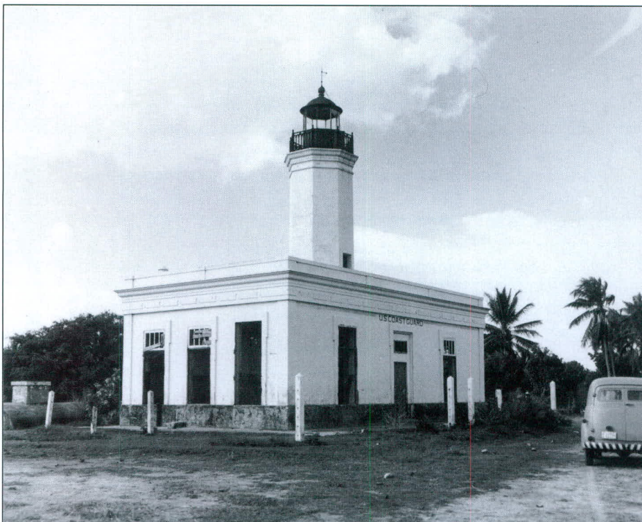
Point Figuras (or Pt. Figuero) was constructed in 1893 on the south shore of Puerto Rico and is typical of most PR lighthouses with a duplex quarters surmounted by the tower. Circa 1955, U.S. Coast Guard photo.
