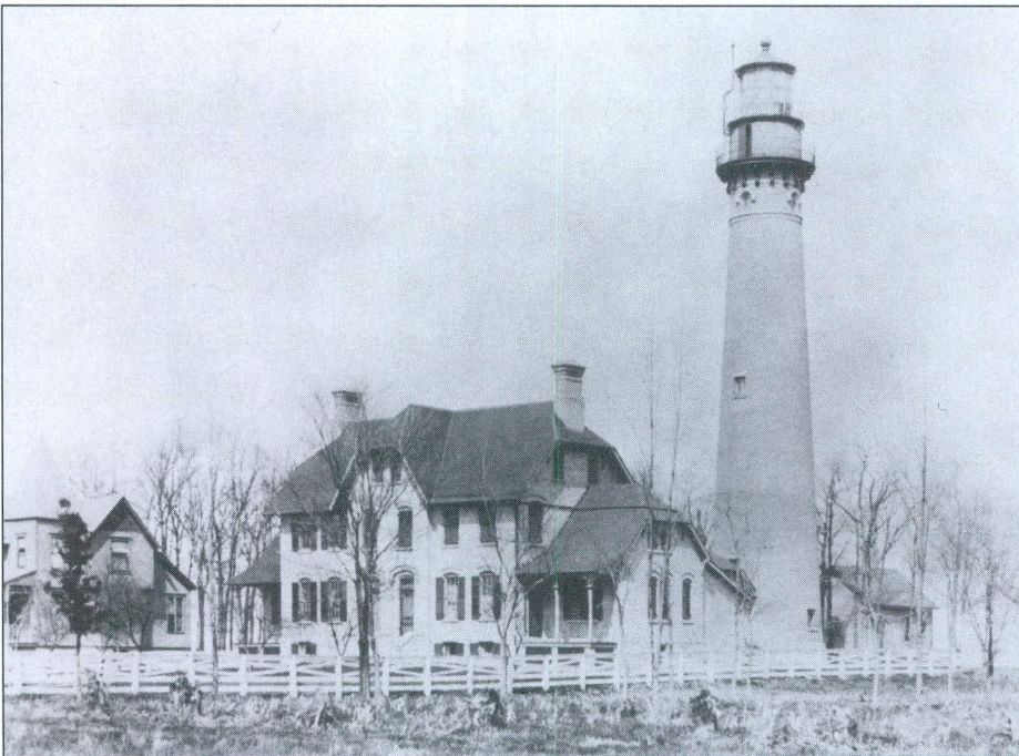
Grosse Point Light Station shortly after completion. The house is a duplex and the small structure immediately to the right of the tower is the fog signal building. Photo courtesy of the Grosse Point Lighthouse.
