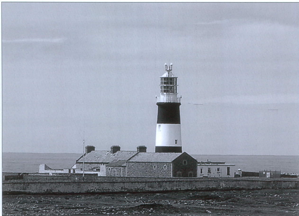
The Tory Island Lighthouse.
