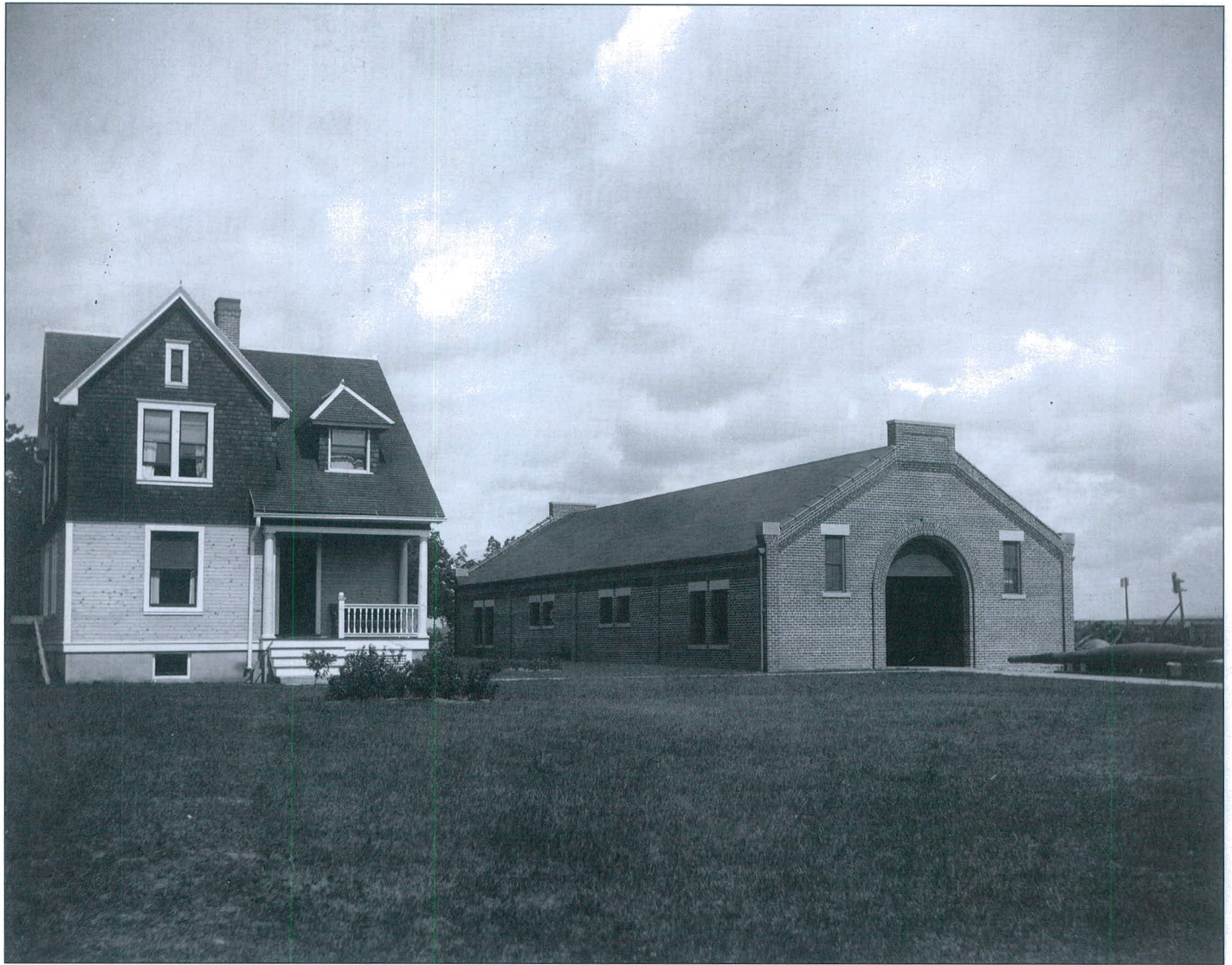
The Charlevoix Buoy Repair and Storage Depot and the custodian's dwelling circa 1914. Photo from the author's collection.
