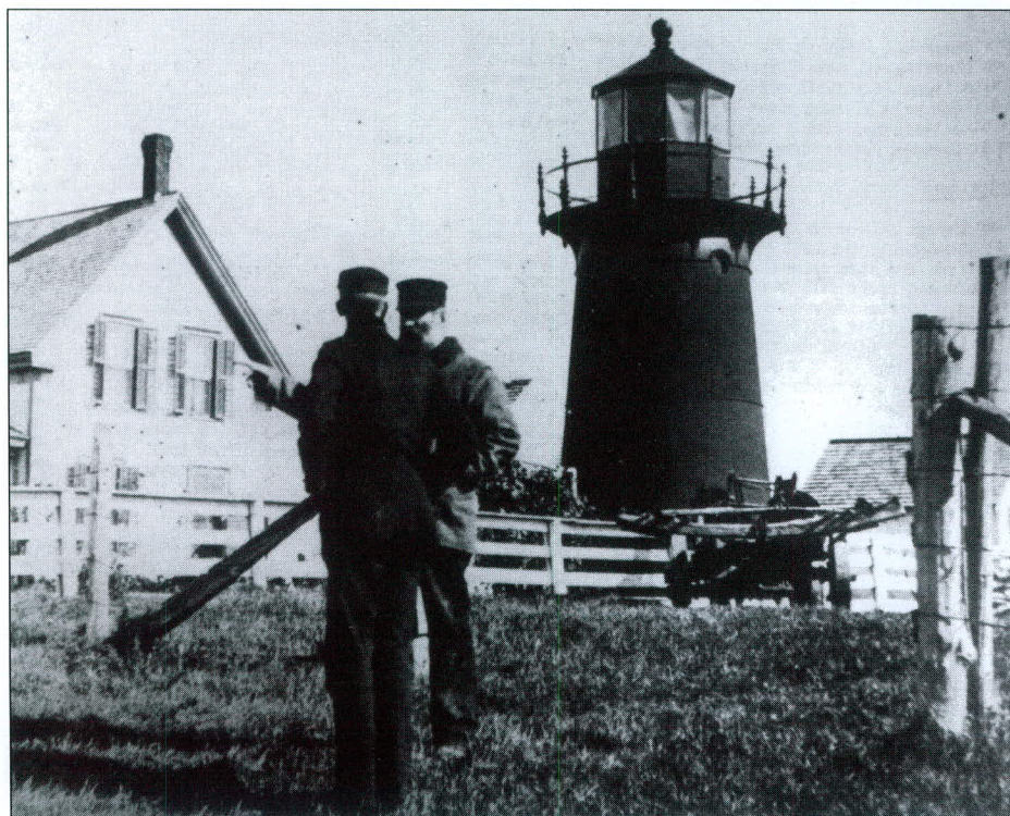
Above and left—The Isle La Monte Light Station showing very little change between the late 19th century (left) and the late 1980s (above). The station was established in 1857 and reconstructed in 1880. The original color of the tower was red; it's now a very unighthouse-like pink. The tower is a generic cast iron tower found at many areas of the country (Cape Neddick, ME; Nobska, MA; Jeffery's Hook, NY; etc.). Top photo by Keeper Elliott Tayman. Left photo courtesy Special Collection, Feinburg Library, SUNY, Plattsburg. In the left photo, note the linen curtains of the lantern have been drawn.
