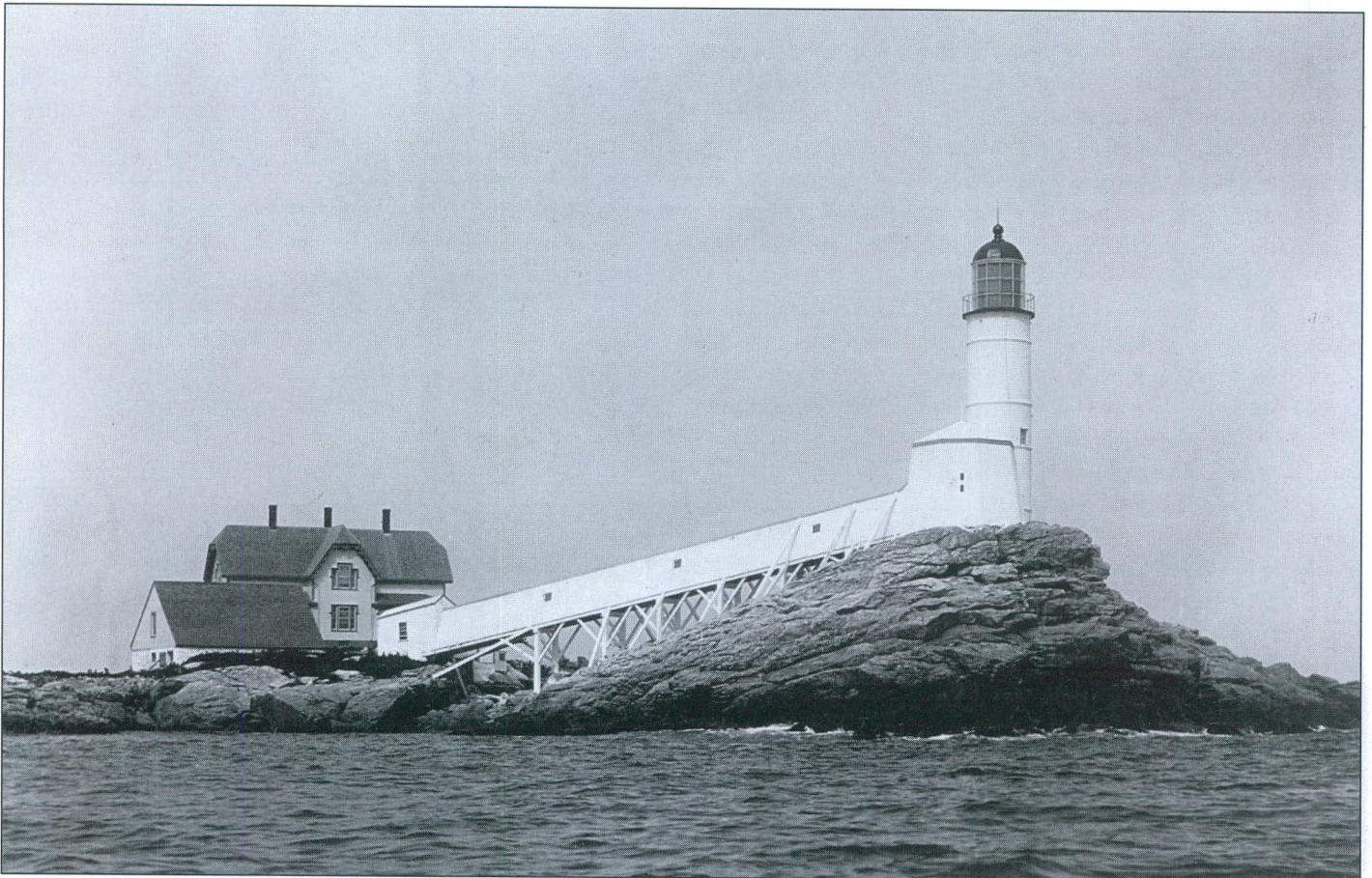
Isle of Shoals showing the 200-foot-long covered walkway, which still exists, and the fog signal building. Photo courtesy of U. S. Coast Guard.
