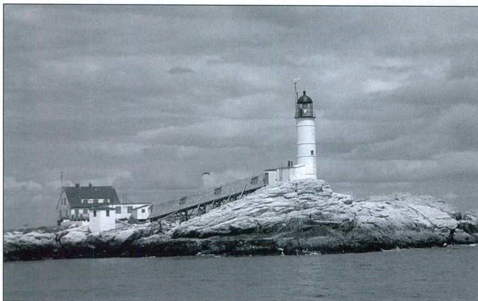
Isle of Shoals Light Station in 1990 showing the Coast Guard-erected dwelling. Photographer unknown.
