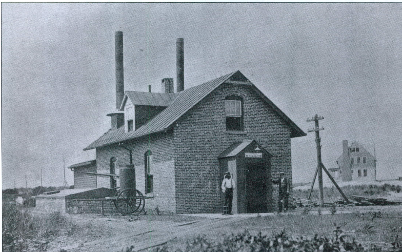
The electric power house at Sandy Hook, NJ furnished the electricity for the Gedney's Channel buoys. Photo from the 1893 Lighthouse Board Annual Report to Congress.
