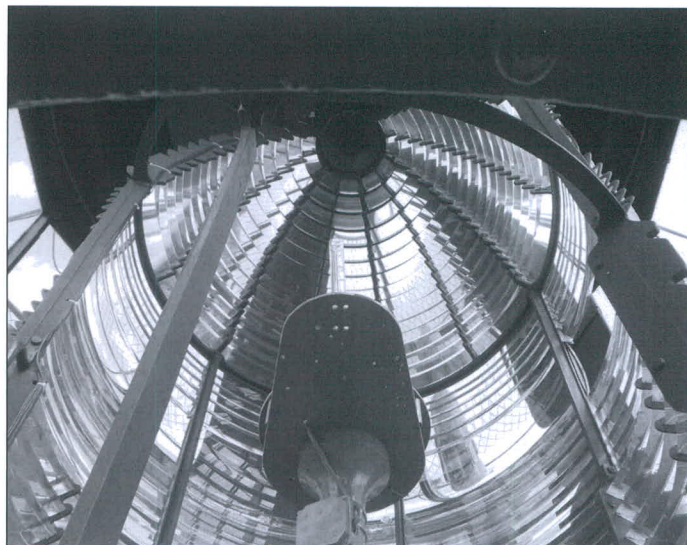
Above left: The original second-order lens still operates and is constantly monitored by the naval base in Szezecin. Eclipsing screens produce a group-interrupted flash characteristic. Two of the screens can be seen in the photo at right, outside the lens.
