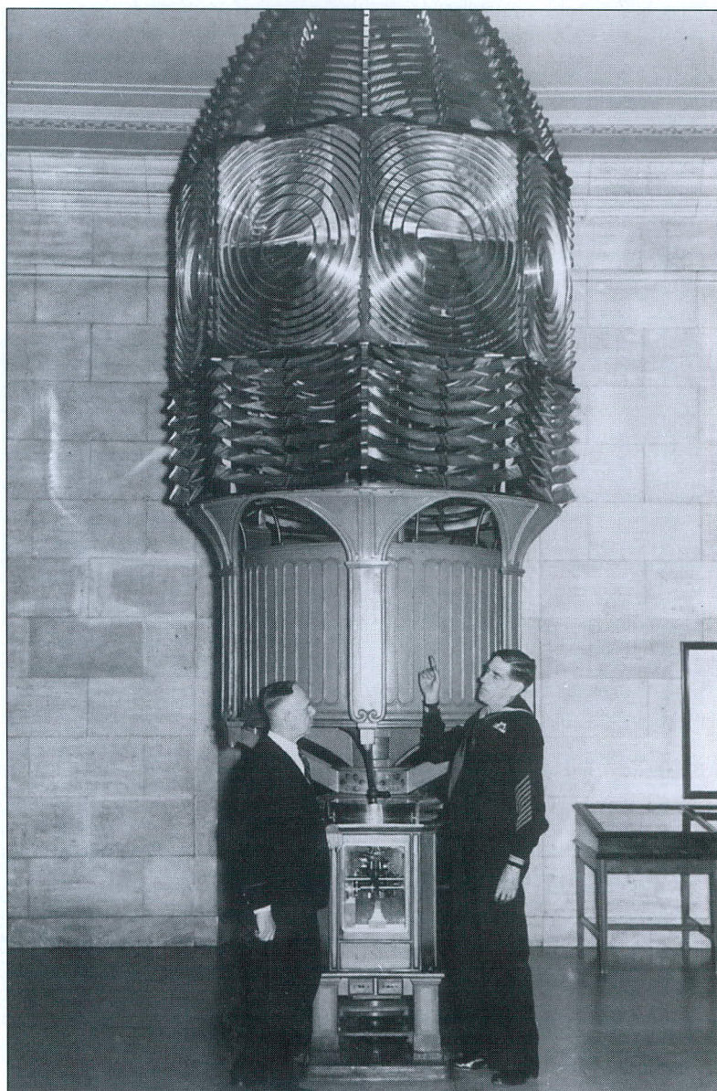
Below – Fire Island's 1st order lens at the Franklin Institute in Philadelphia. Note the clockworks in front of the lens. This lens is a duplicate of the Farallon Island, California lens. Photo courtesy of the National Park Service.
