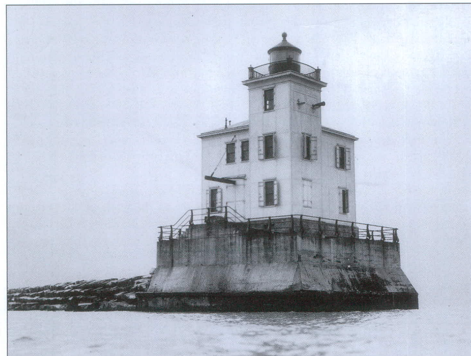
The new steel-walled West Breakwater Lighthouse was the pride of Fairport when it went into service in the summer of 1925. The lantern had a fourth order lens that flashed white every three seconds. The dwelling was spacious, but the air diaphone foghorn, seen projecting from the upper portion of the tower, probably made for many sleepless nights. Photo from the U. S. Lighthouse Society archives.
