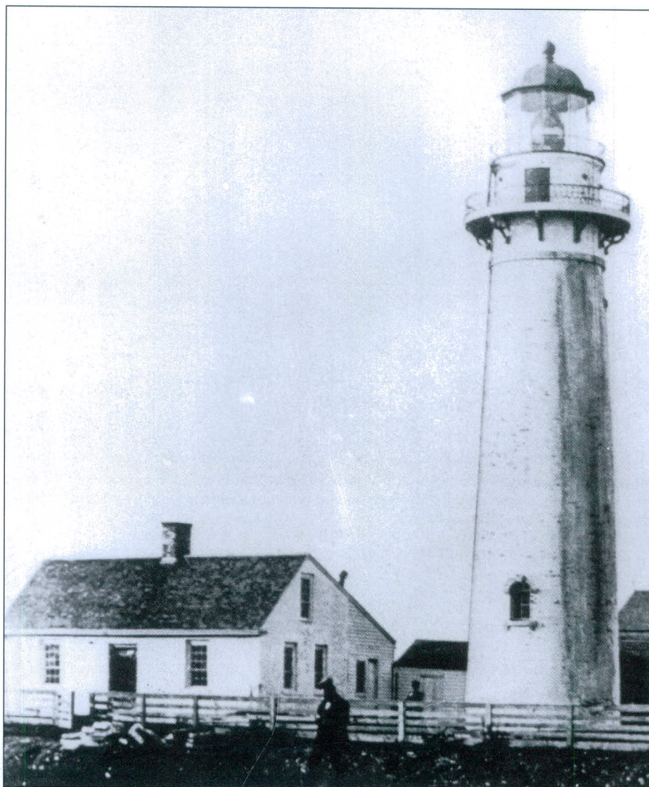
The original brick lighthouse and saltbox dwelling, built in 1825 by New England native Jonathan Goldsmith, looked sturdy enough, but within a decade problems arose with the foundation. Eventually, the station was completely rebuilt. Photo courtesy of Fairport Marine Museum.
