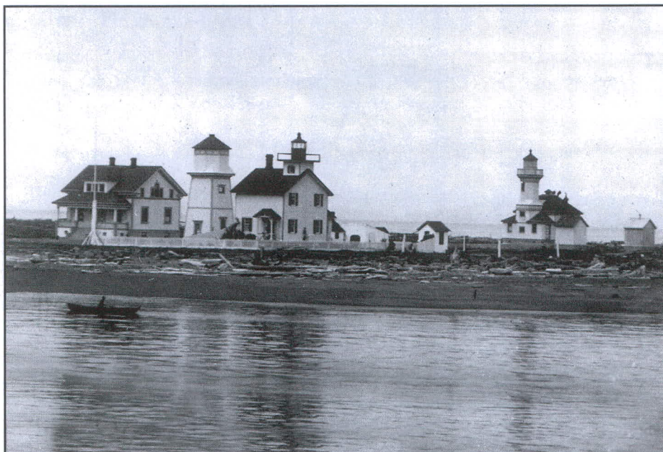
The Ediz Hook Light Station in transition. From left are the Leick-designed new keeper's dwelling, water tower, original lighthouse, storage sheds, new lighthouse and oil house. The old lighthouse is thought to have been moved to Port Angeles, without the lantern room, and used for various things. It is speculated that the building, below left, is the original lighthouse.
