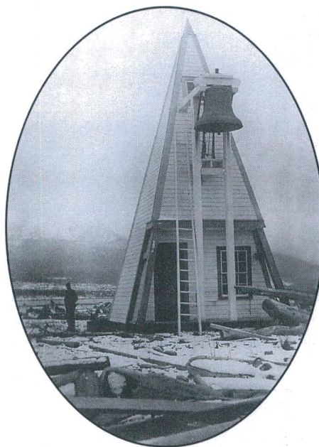
The 1885 fog signal building in 1907. A descending weight inside the tower powered an automatic fog bell striking mechanism that periodically struck the bell with a hammer. The 1890 Light List states, "... struck by machinery every 15 seconds. At times this bell cannot be heard over one-quarter mile." Photo courtesy Bert Kellogg Collection, North Olympic Library System.
