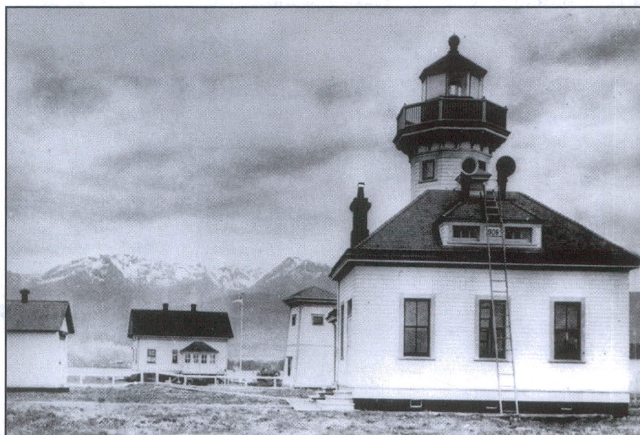
Right – The new Ediz Hook station, which was constructed in 1908. From left are the oil house, keeper's dwelling, water tower (which has been reduced in height) and combination lighthouse-fog signal building. The fog signal horns can be seen protruding from the roof. This second Ediz Hook lighthouse was sold and moved to Port Angeles, above right.
