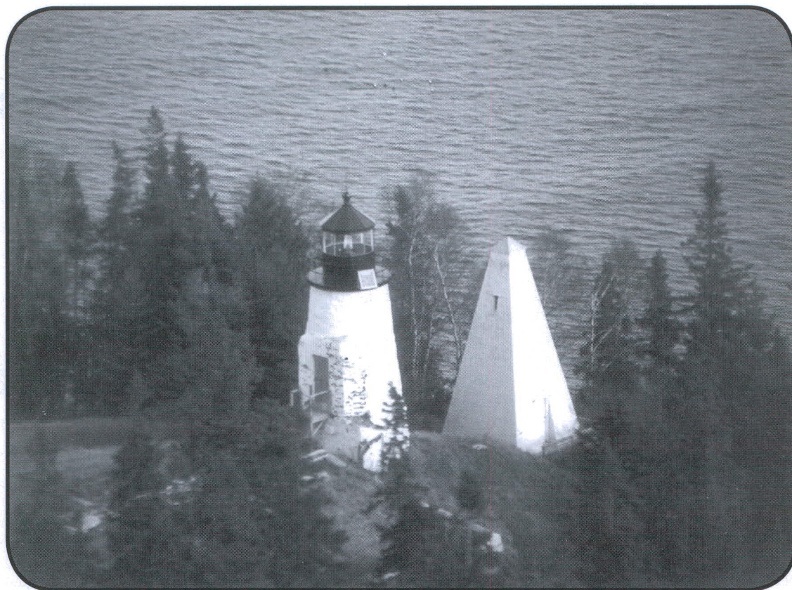
The tower of the Eagle Island Light Station. One can see where the walkway to the house was attached. The fog bell building at right was added between 1908 and 1915. 1990 photo. Photographer unknown.
