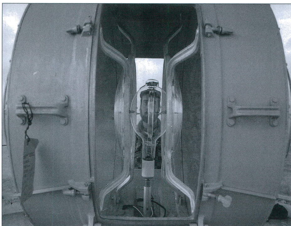
Above and below – Interior view of a DCB-36 showing the 1,000-watt mercury vapor lamp, used in Canadian lighthouses, and the doublet lenses on either side. Photos courtesy of Chris Mills.
