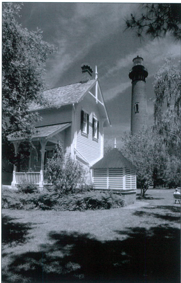
The small structure to the right of the keepers' house is a cistern. Rain water was gathered from roof runoff and directed through pipes to a cistern on either side of the house to provide fresh water for keepers' families. This technique of water storage was standard for all American lighthouses until the mid-20th century.
