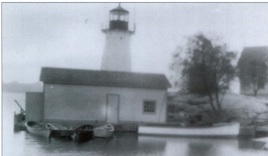
Boathouse built in 1920 by Keeper Hill. Ralph Hill photo.
