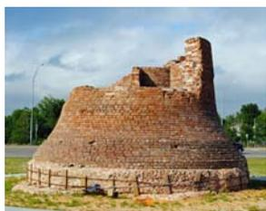
The City of Pascagoula has completed the initial restoration of the Round Island Lighthouse, which was moved from offshore to the city. The USLHS Gulf Coast tour in 2011 visited the base of the light from which the tower rose again, using bricks from the original structure. They continue to raise funds for further work and now have a Society stamp. We
