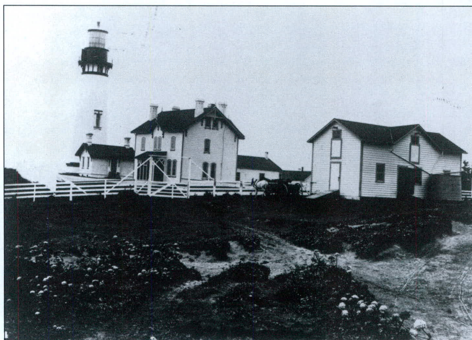
The large building at right is the barn. Note the water cistern to the right of the barn door, water was collected from the roof. Oregon Historical Society photo.
