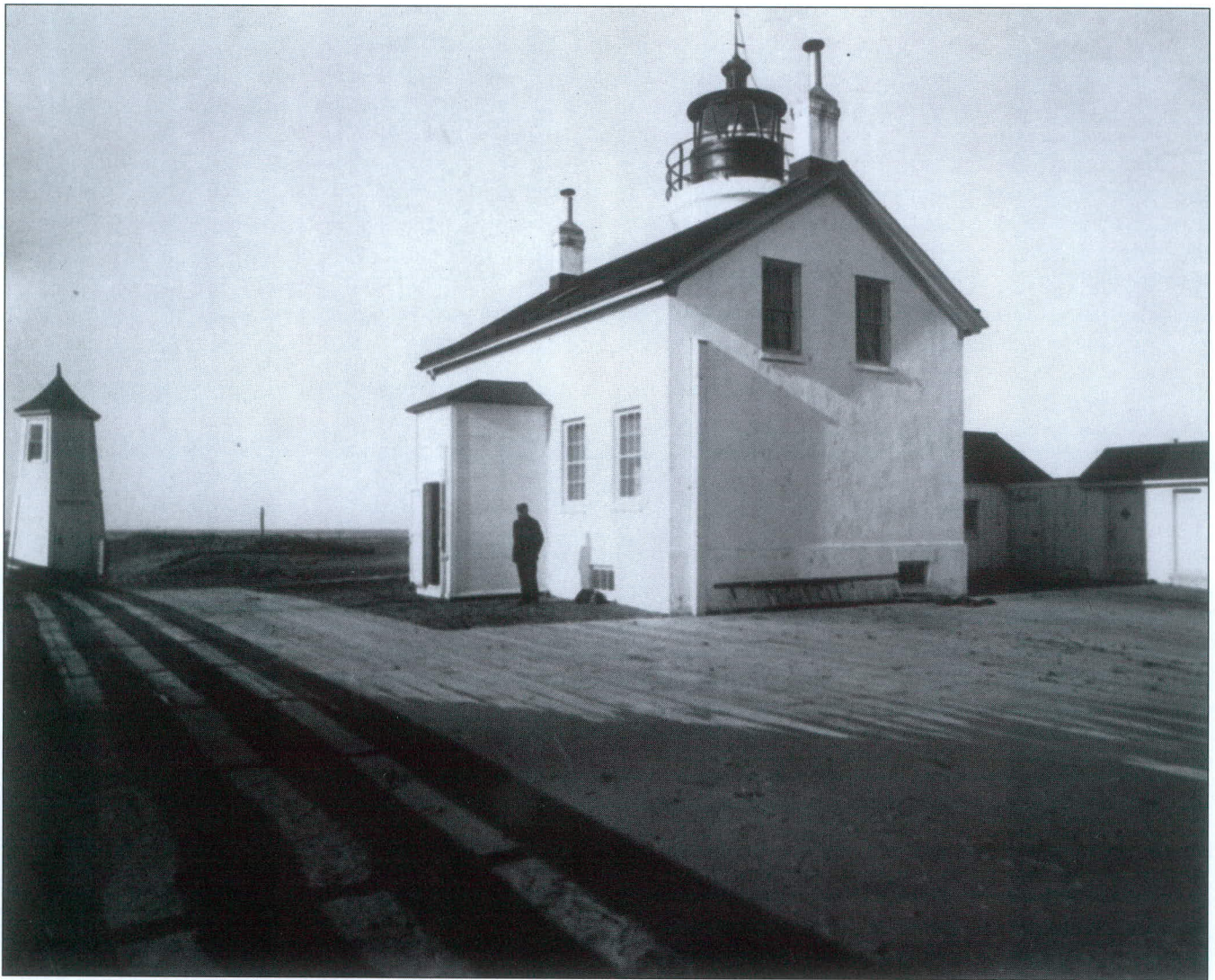
Cape Shoalwater Lighthouse circa 1930 looking northeast. The small structure at left is apparently some sort of a lookout. Perhaps to watch vessels crossing the dangerous bar. U.S. Lighthouse Society photo.
