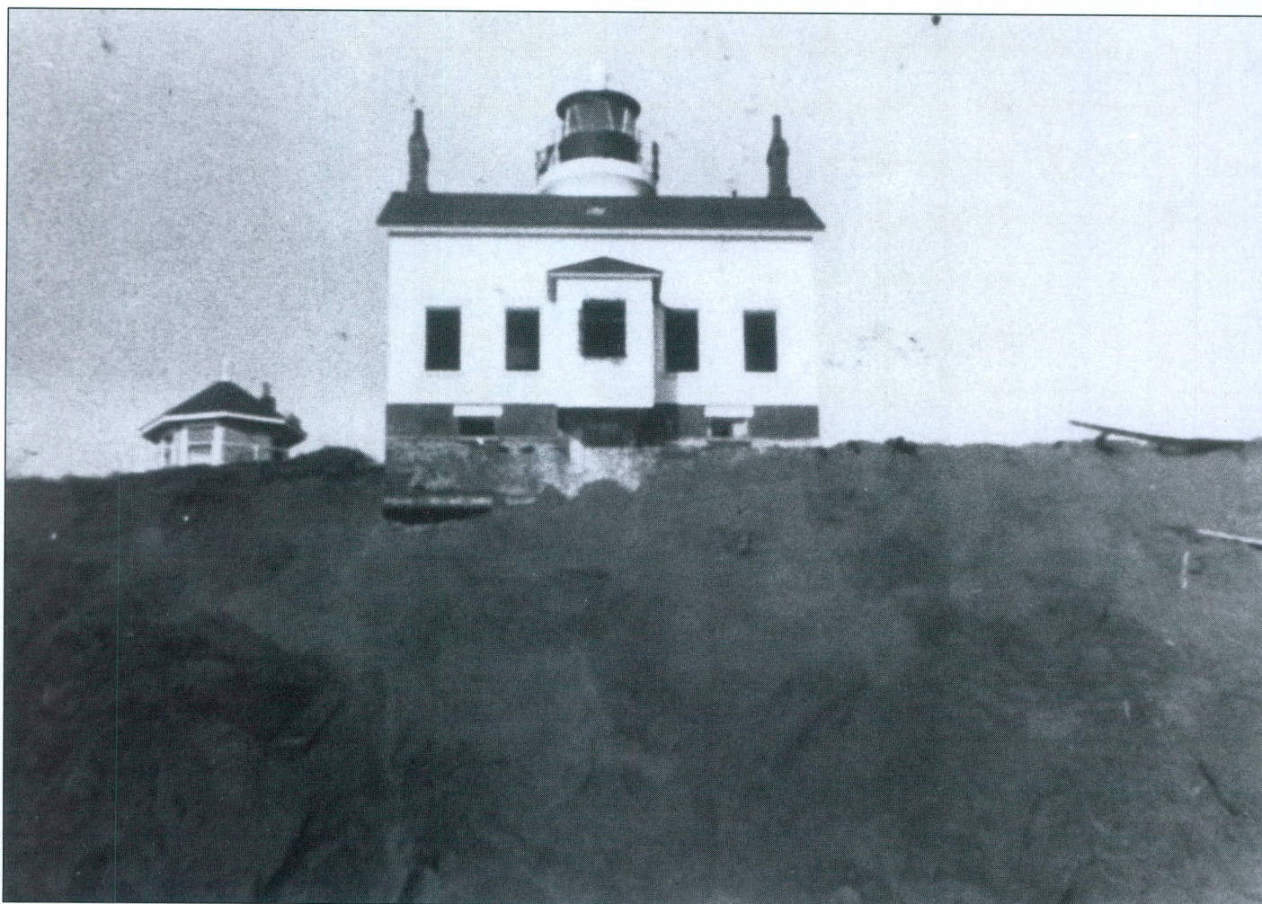
The lighthouse is seriously endangered by erosion in this photo with most of the foundation exposed. The small structure at left appears to have been moved back from the eroding dunes. Photo courtesy of Ainsley Dixon, late 1930's.
