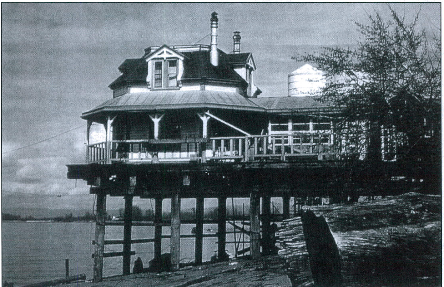
Above – The Willamette Light Station after it was relocated near Portland and used as a pilot office. U. S. Lighthouse Society photo.
