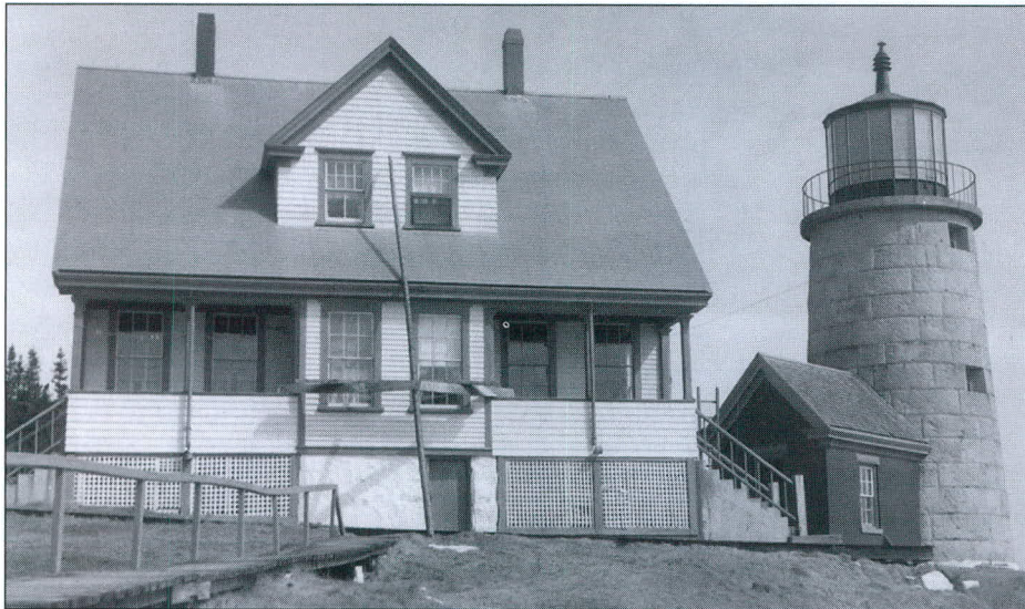
The "new" Whitehead Island keeper's dwelling, possibly in the 1920's. Note the crude scaffolding indicating that the house had just been painted. U. S. Lighthouse Society photo.
