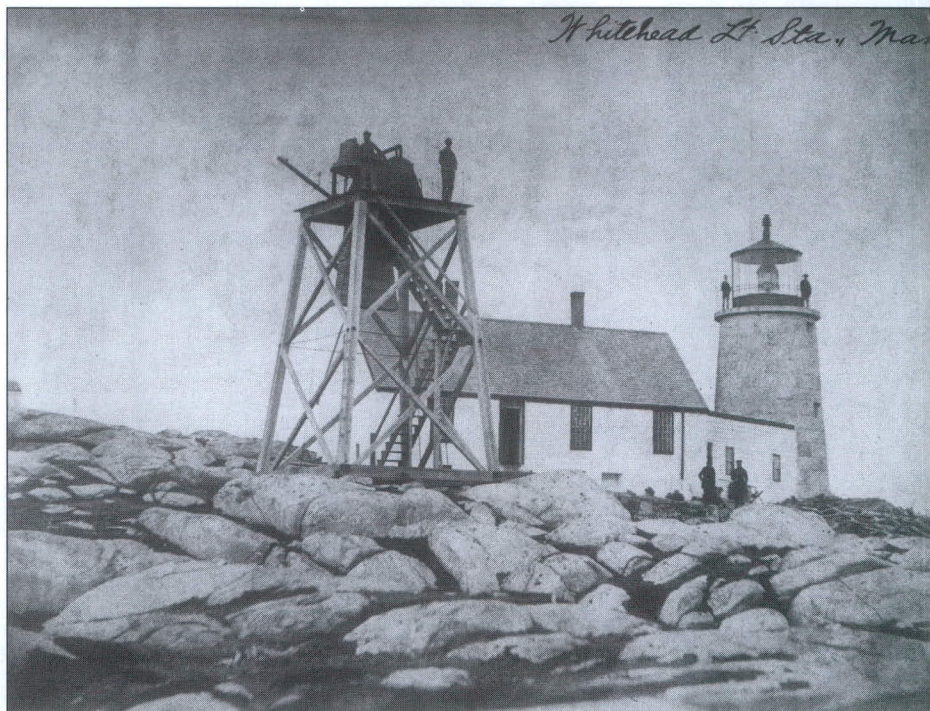
The 1853 two-story wooden tower and bell fog signal. The bell was struck by an automatic striking mechanism. Photo courtesy of the author.
