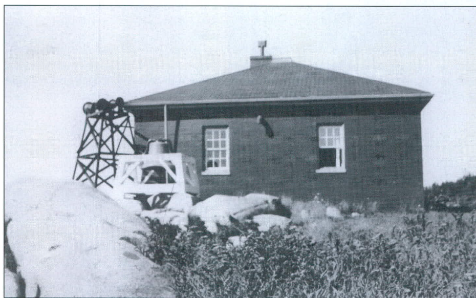
The 1871 whistle house. Note the multi-directional fog signal horns on the skeleton tower and the standby bell signal. Photo courtesy of the author.
