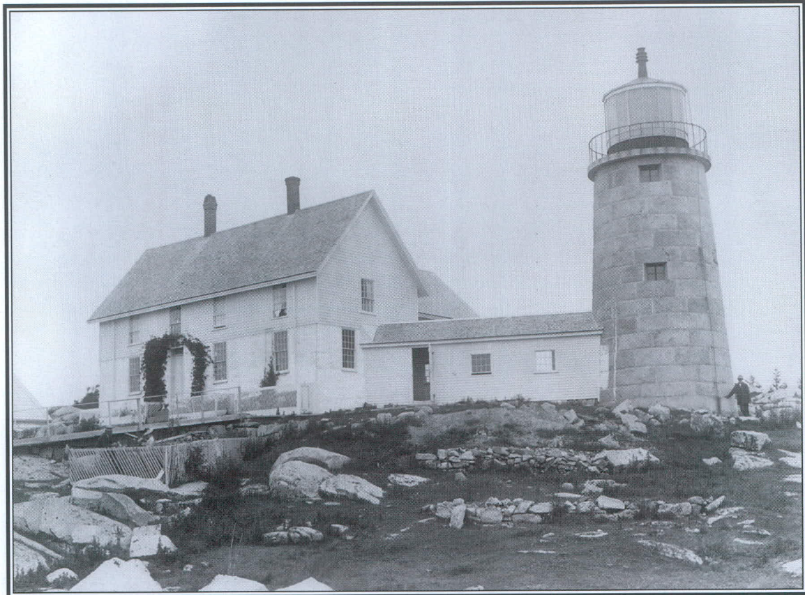
Whitehead Light Station after a wooden second story was added to the original one story stone house. National Archives photo.
