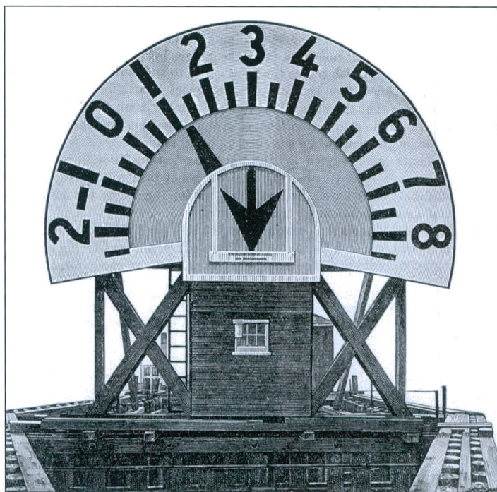
The Tidal Indicator on Reedy Island in the Delaware River. Photo courtesy of NOAA.
