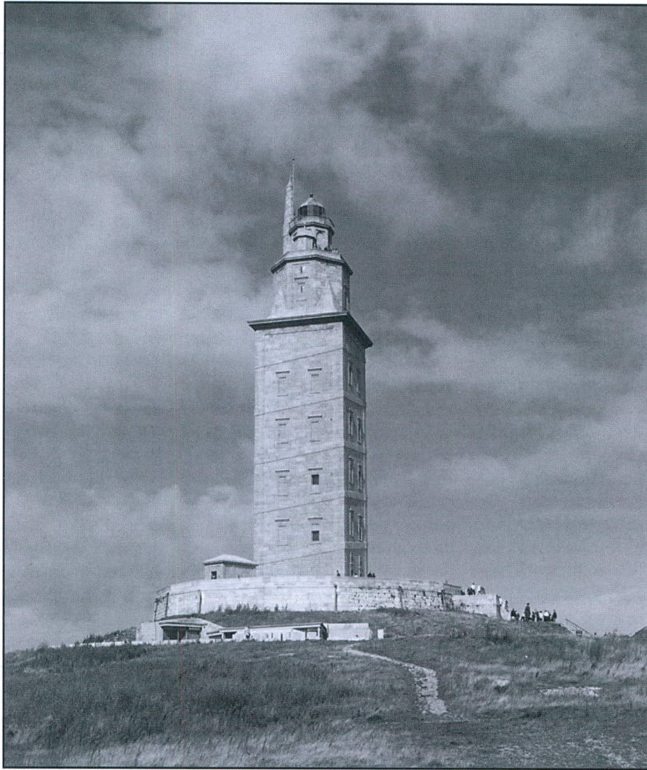
La Coruña, the oldest operational lighthouse in the world, constructed by the Romans. It's also known as the Tower of Hercules. The tower is 159 feet high and originally had an open fire on top as the illuminate. An 1899 Light List states that the tower was altered in 1847, 1861, 1872 and 1898. Author photo.
