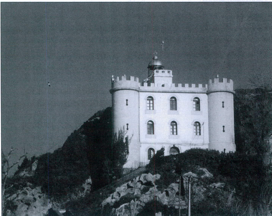
Faro de la Plata lighthouse, resembling a castle. It is also listed in some Light Lists as the Port Pasajes Lighthouse. It was constructed in 1855 and still contains a 4th order Fresnel lens displaying a fixed white light. Photo by the author.
