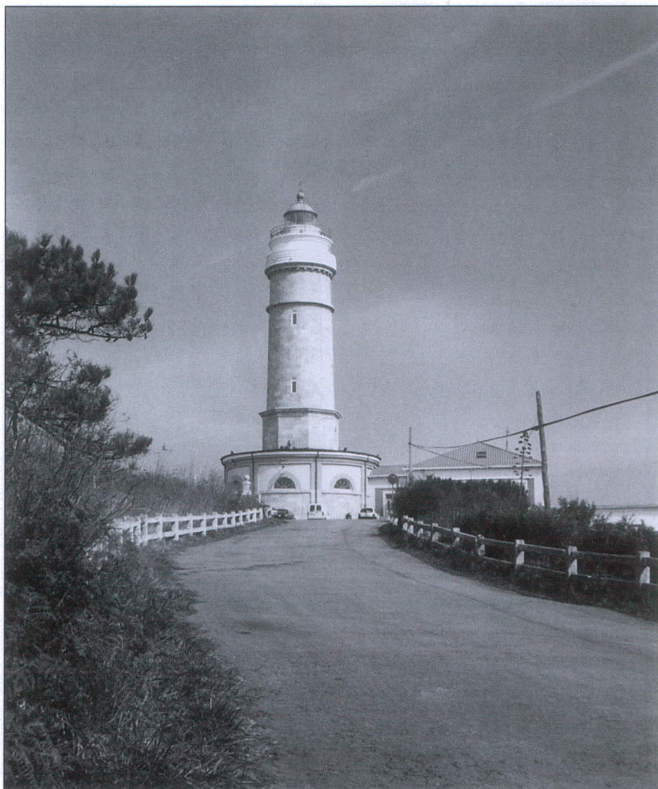
Above and below — the Cabo Mayor lighthouse which was constructed in 1839. A turn of the century light list calls it the Santander Lighthouse. The tower is 98 feet high and is located 298 feet above sea level. The original 2nd order lens has been replaced by a 3rd order lens. Photos courtesy of the author.
