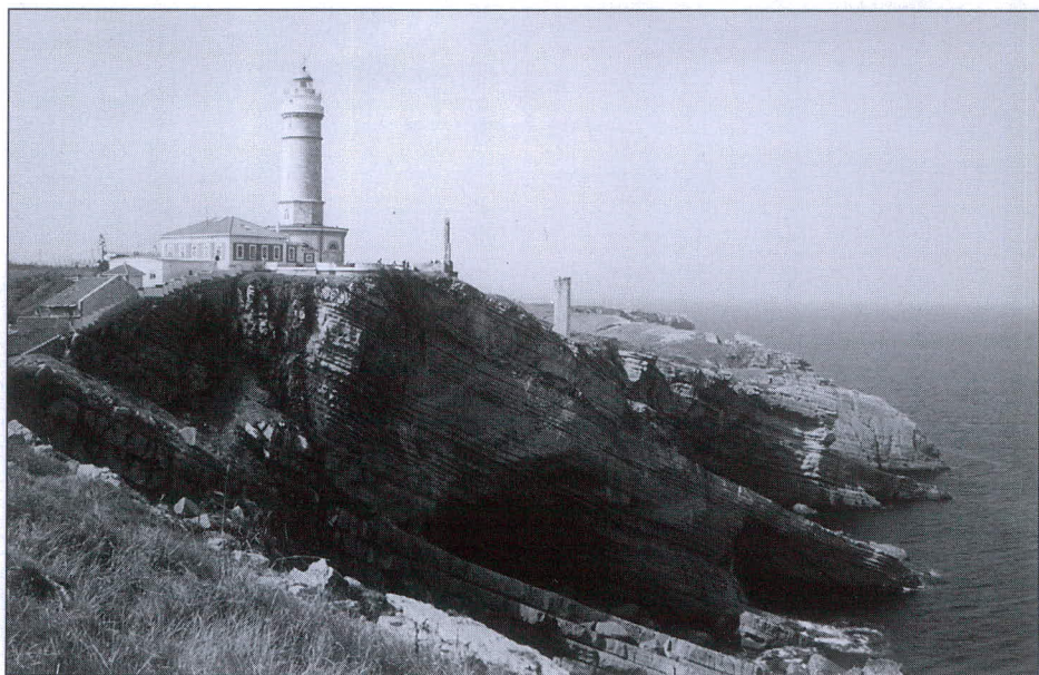
Above and below — the Cabo Mayor lighthouse which was constructed in 1839. A turn of the century light list calls it the Santander Lighthouse. The tower is 98 feet high and is located 298 feet above sea level. The original 2nd order lens has been replaced by a 3rd order lens. Photos courtesy of the author.
